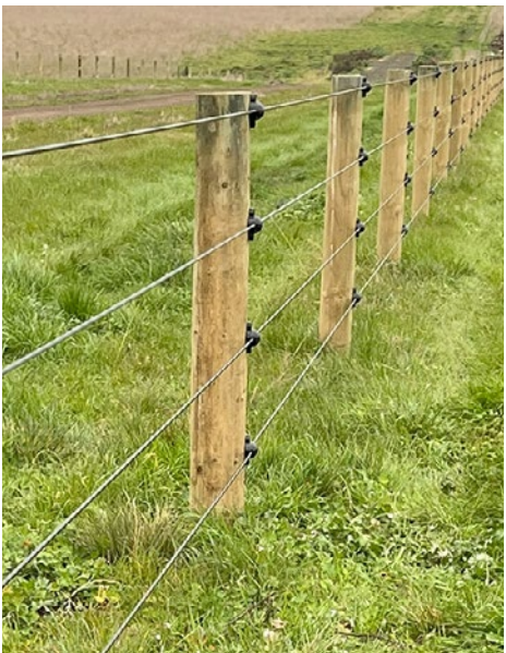
Post and Wire Fencing
