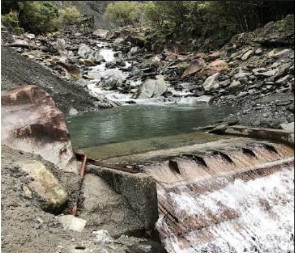
Figure 3: Example of a Tyrolean weir (Source: Stantec, 2025).
