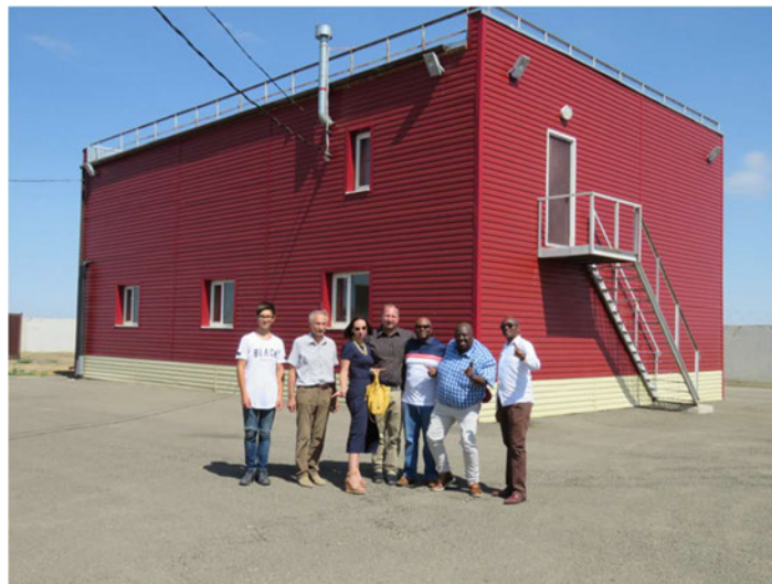
Figure E-2: Shows the outside of a 600 000 m 3 /day Residential and Commercial WWTP Module in Krasnodar Territory. The Development team are also shown in the picture.
