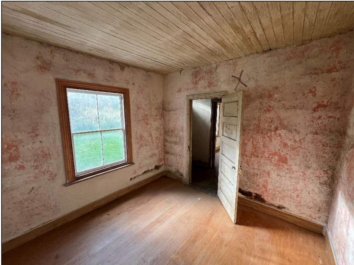
Photo 10 Monitor any damp patches inside
