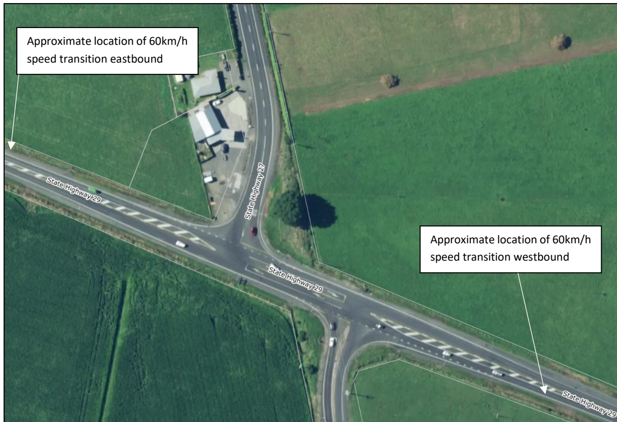
FIGURE 5: SH27/SH29 INTERSECTION NORTHEAST OF SITE
