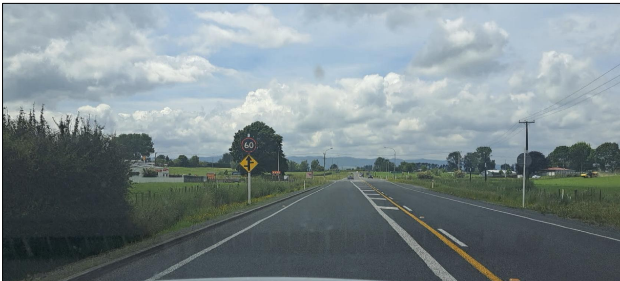
FIGURE 6: VARIABLE SPEED SIGN ON SH29 – WESTERN INTERSECTION APPROACH
