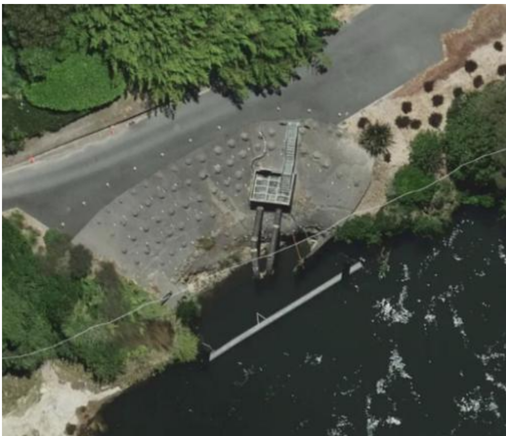
Figure 3: HCC intake on the Waikato River.
