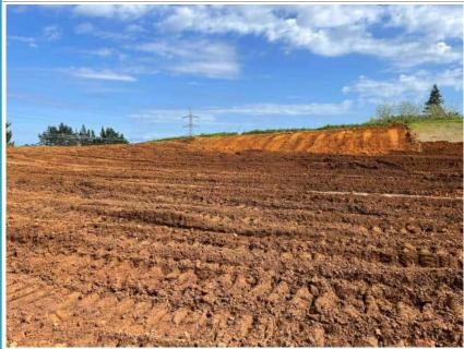
**Looking south** – Cutting of A4 comprising clayey silt material with basalt clast inclusions.
