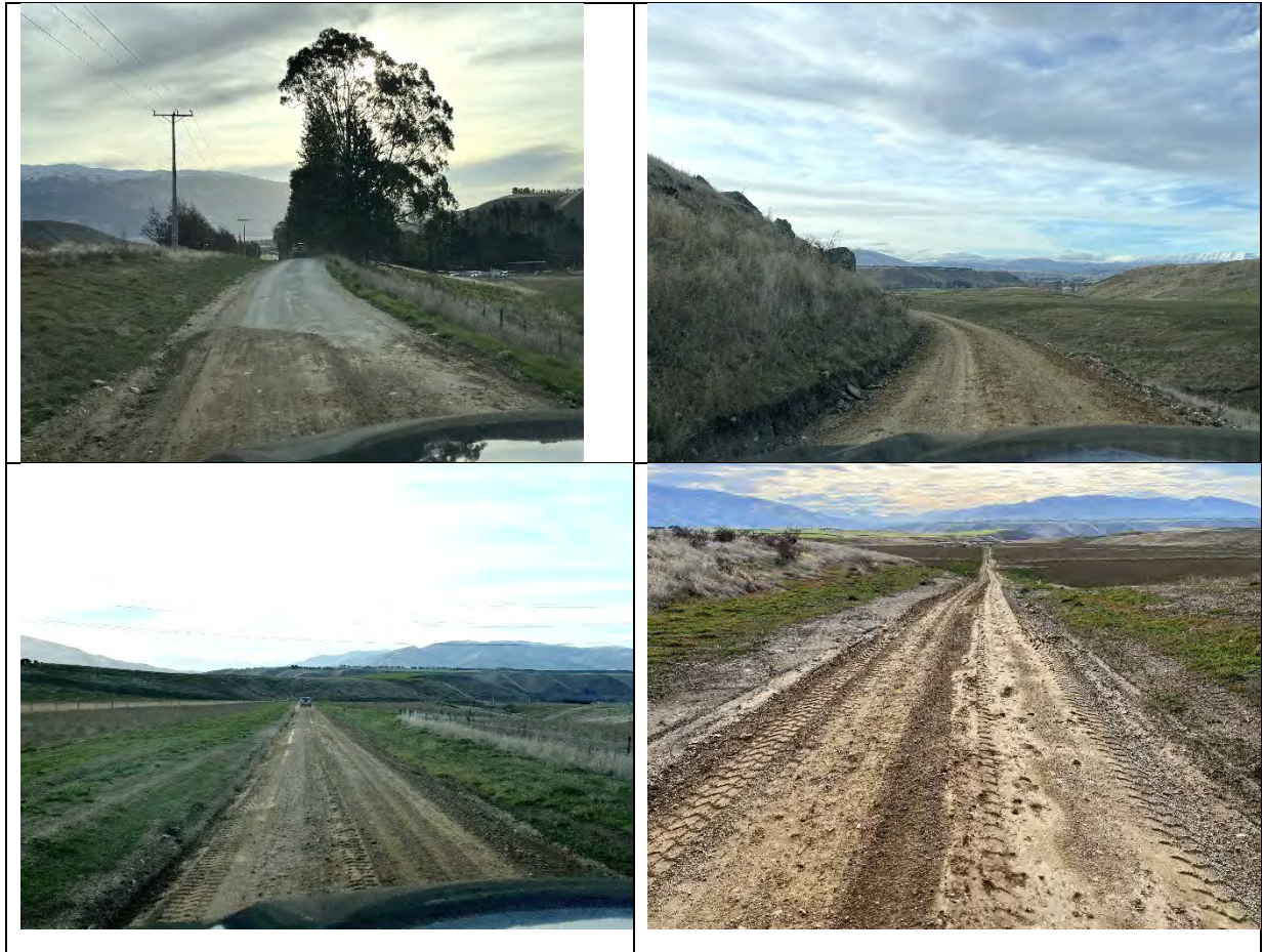
Figure 3-9: Thomson Gorge Road (Ardgour Road to Matilda Rise)
