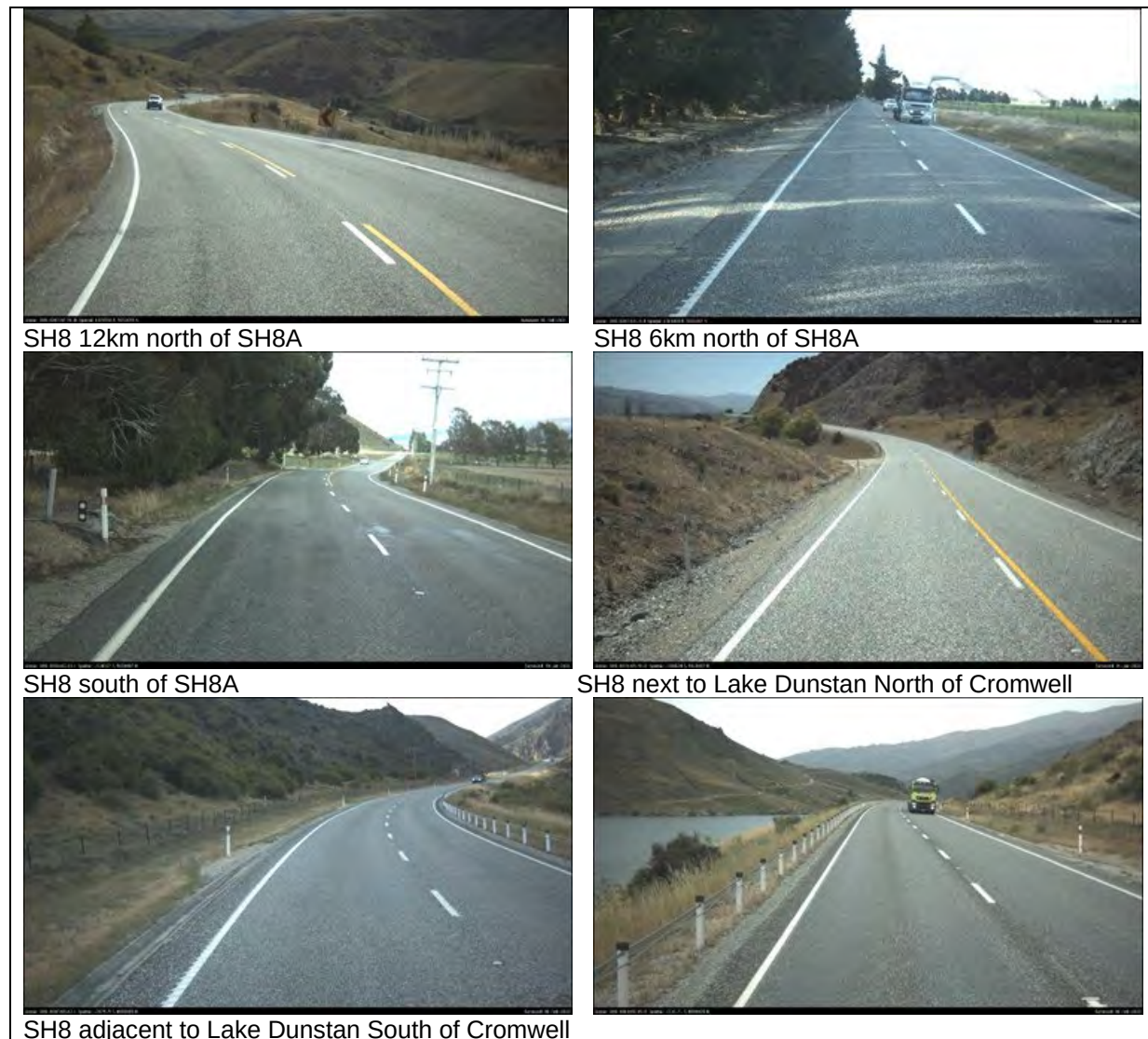
Figure 2-1: SH8 Typical Photographs
