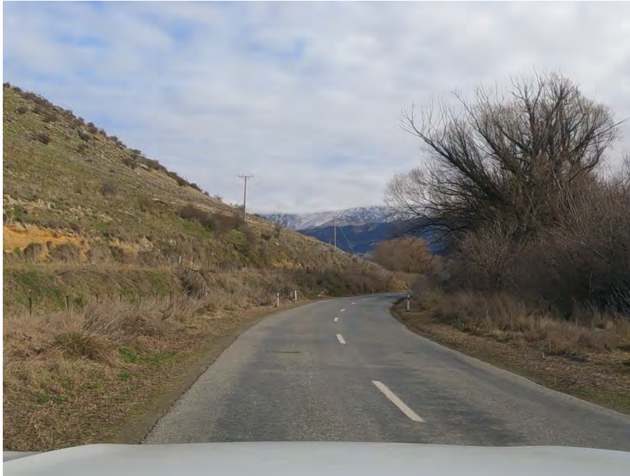
Figure 3-2: Ardgour Road – Curve 0.4km South of SH8
