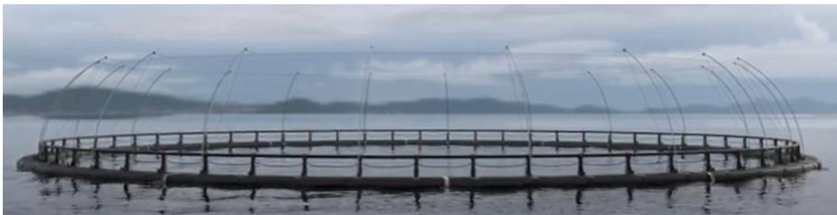
Figure 6-4: Example of circular pen with jump fence and bird netting (Source: AKVA Polarcirkel 500R plastic pens)
