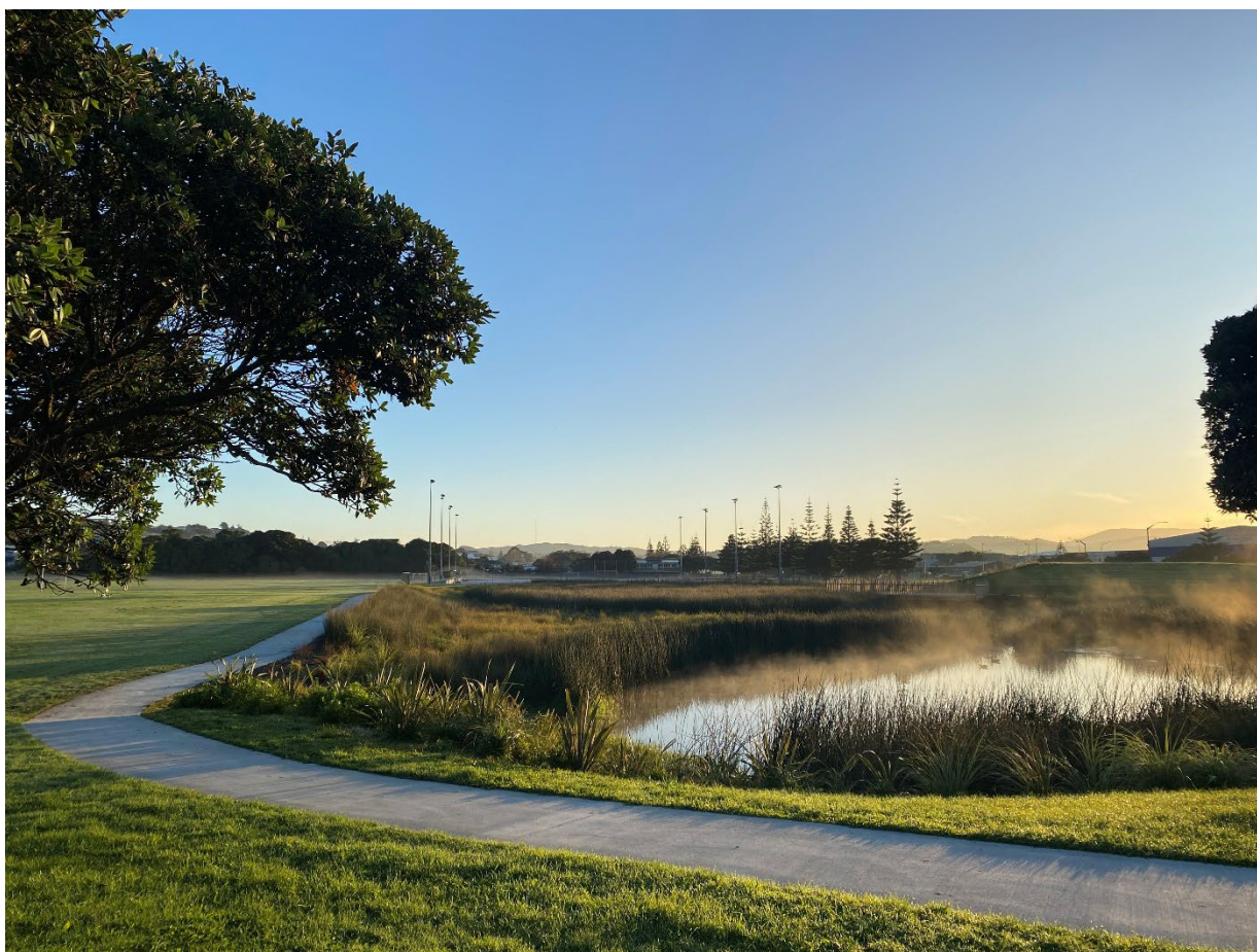
Figure 1 Constructed stormwater wetland with forebay to the right of path
