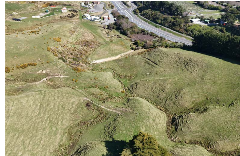
Existing Valley Conditions
