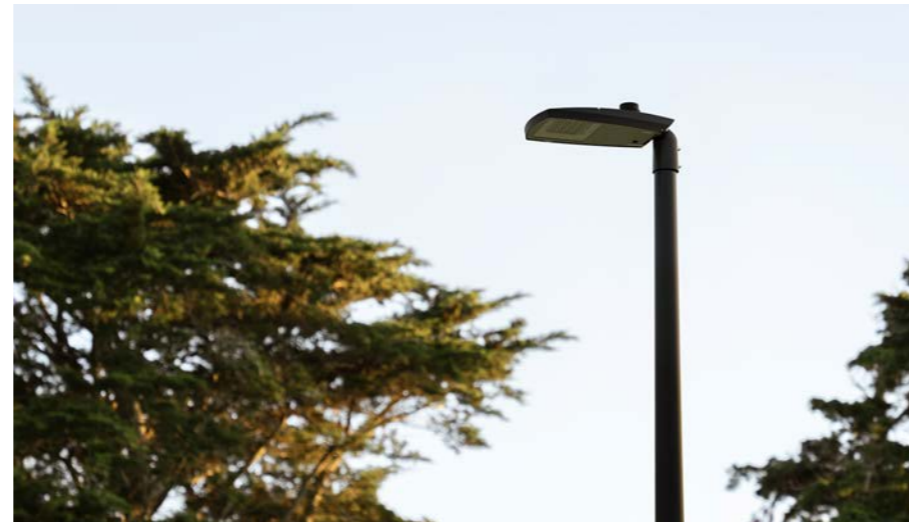
D2 Carpark + pathway light: SHS Column - Nox luminare
