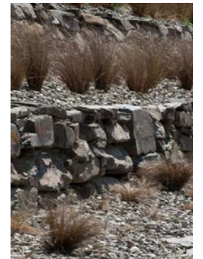
E8 Streamside retaining/ rock revetments
