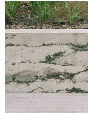
A6 Feature walls (off-form concrete, multi-pour)
