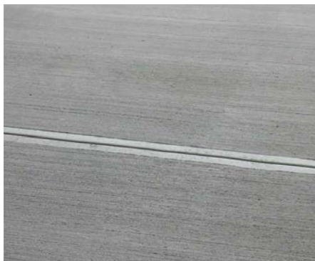
A1 Brushed concrete with a trowelled centre line on shared paths
