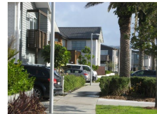
Screened parking integrated into frontages, Hobsonville Point, Auckland. This approach is designed into the housing typologies for MD housing areas.
