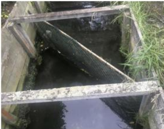
Example of a 'fence' type fish screen.
