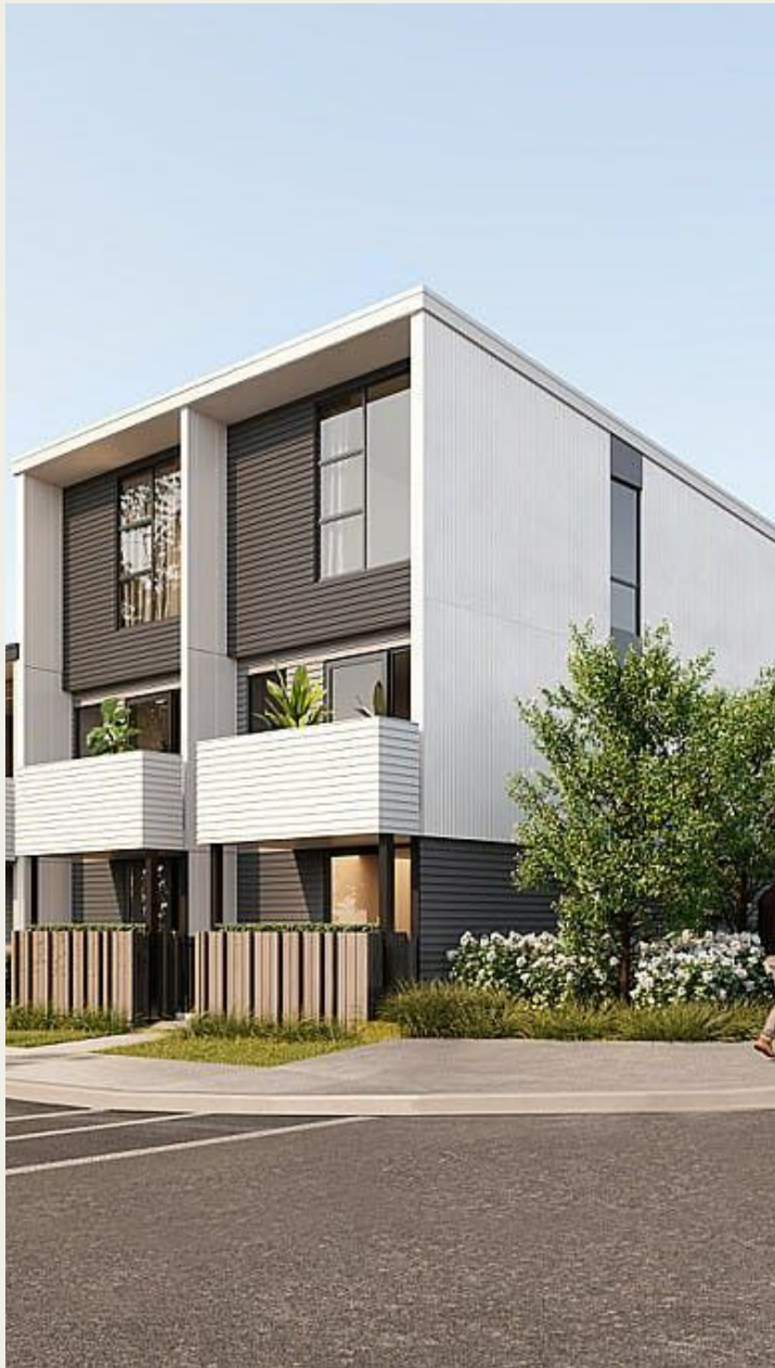
Kapiti Road 78 lot residential subdivision in the heart of Paraparaumu
