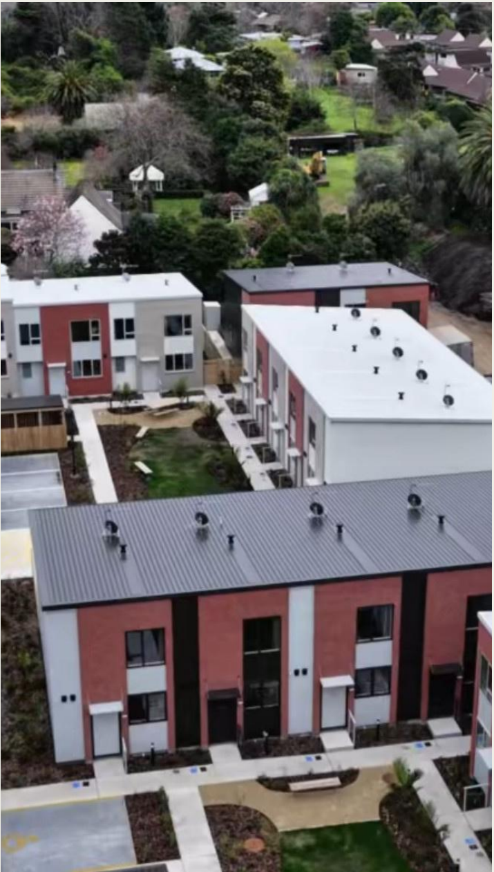
Kainga Ora Partnership Project 26-unit townhouse development in Kapiti, comprising 11 three-bedroom and 15 two-bedroom homes
