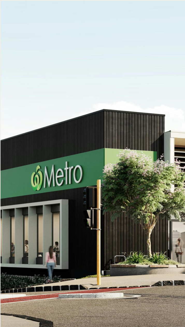
Countdown Metro, Herne Bay Located in the seaside suburb of Herne Bay, the 1683sqm store includes a supermarket retail area, storage and associated offices, with carparking for 52 in the basement
