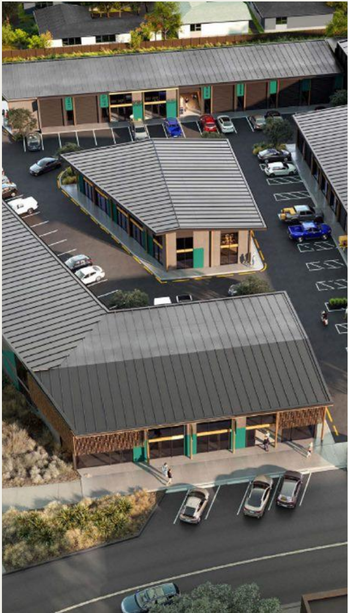
Lyall Bay Junction An industrial-commercial development comprising 56 units. Catering to a wide range of business needs for dynamic small and medium-sized businesses in the beachside suburb of Lyall Bay in Wellington
