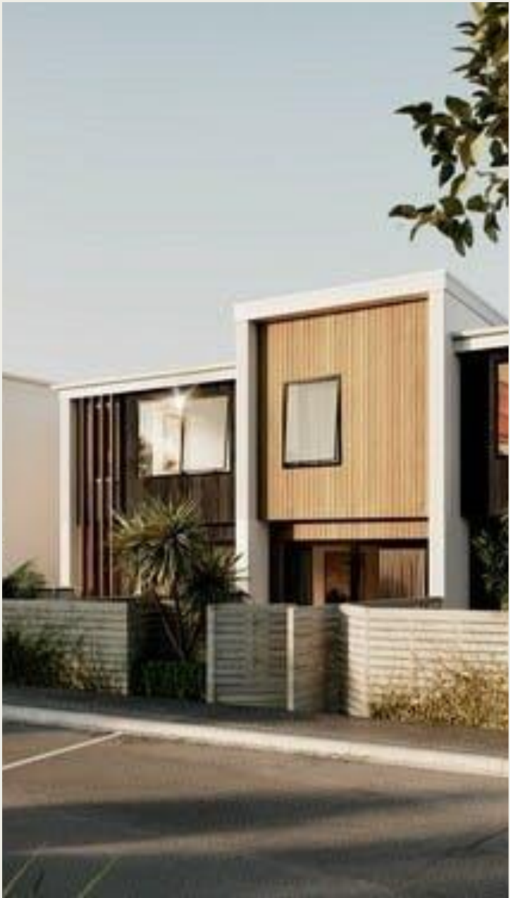
Queens Drive 28 lot residential subdivision located in Lyall Bay, Wellington
