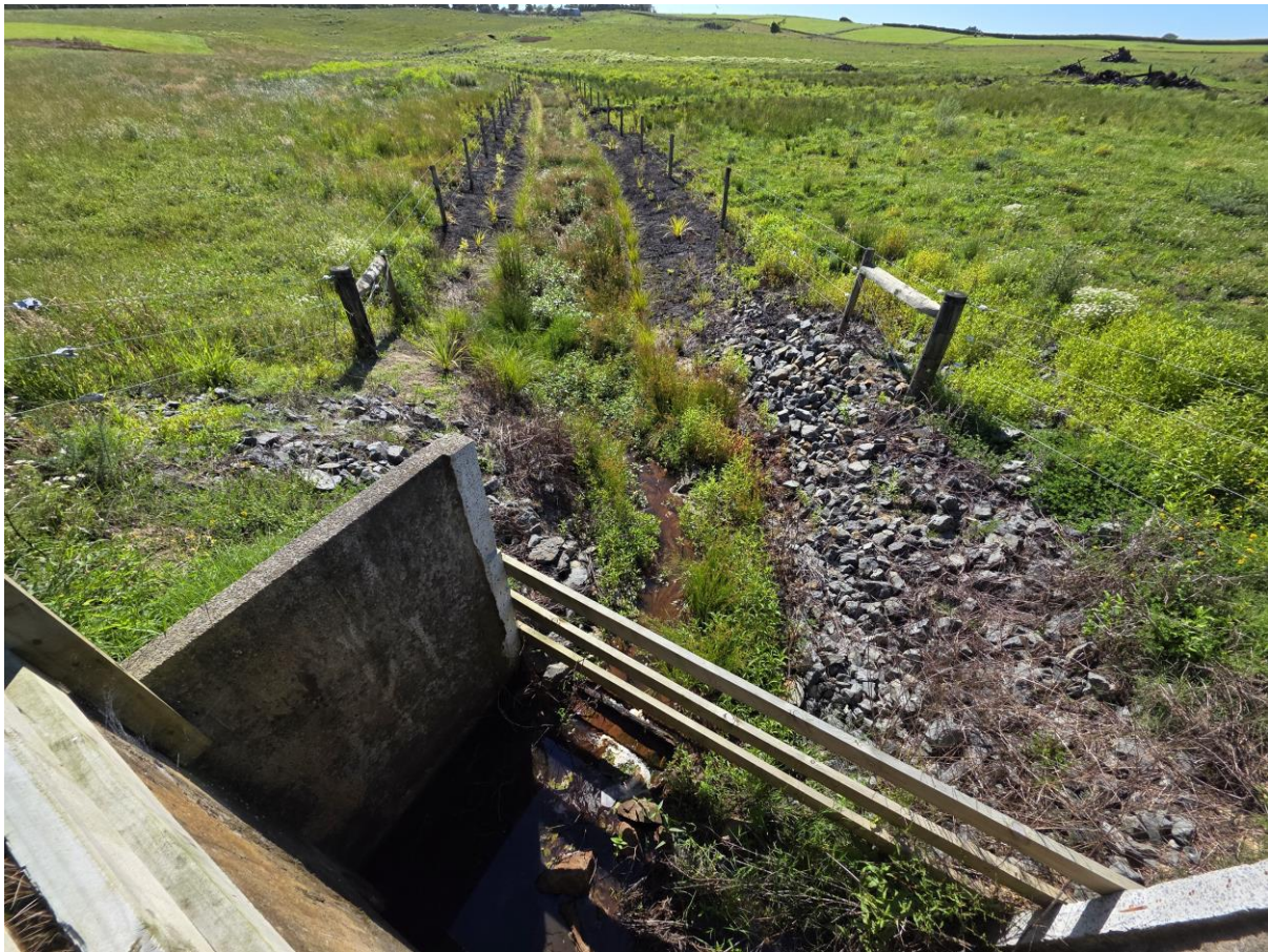
Figure 19. Start of the modern realignment facing east from the corner. A new bridge and culvert have been constructed as well as the new ditch alignment being made wider with more potential to soak.
