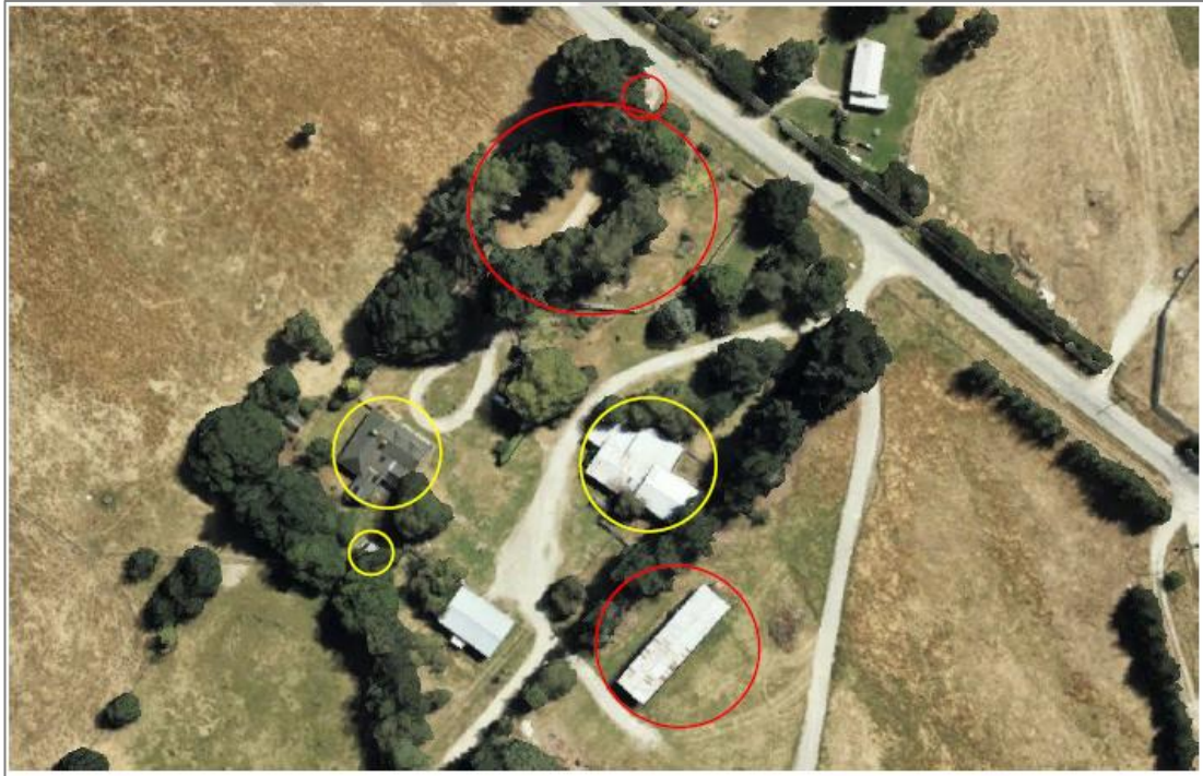
Figure 65: David Jolly's farm buildings indicated in yellow, other structures with historic significance in red (from Figure 6 of the Origin Assessment).
