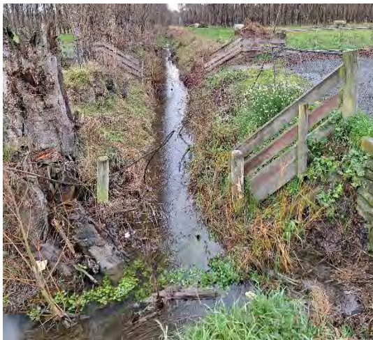
Figure 3-2 McIntosh Drain Near the Motorway Crossing
