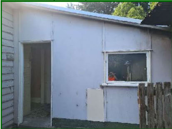
Photo 17 – House extension with PACM cladding
