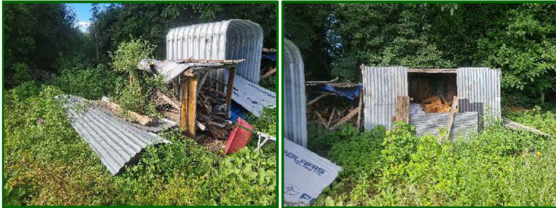
Photo 21 and photo 22 – Scrap material, southern side of pottery workshop
