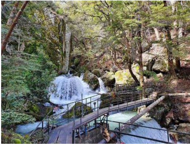
Figure 19: Wye Creek frontal weir intake structure
