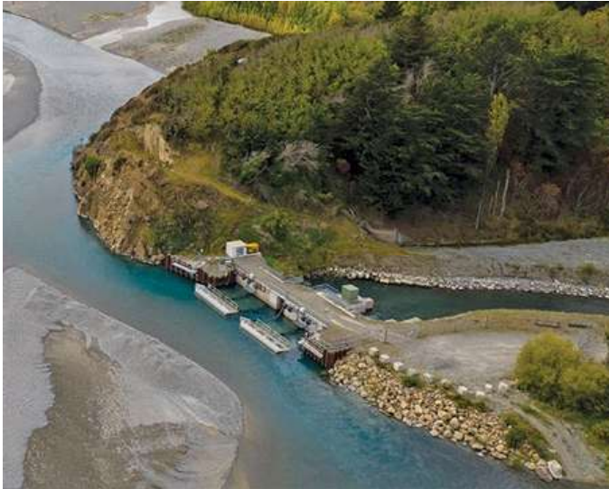
Figure 21: Waimakariri Irrigation - Lateral Intake without weir
