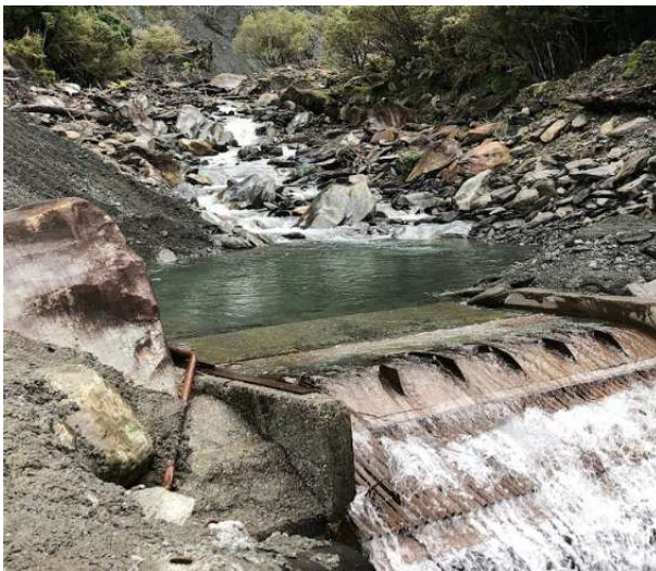
Figure 22: Tyrolean Weir intake - Big Wainihinihi Intake 2, Westland District
