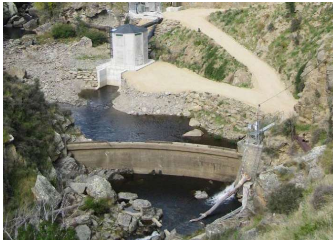
Figure 20: Teviot Irrigation Company – Frontal Weir Intake
