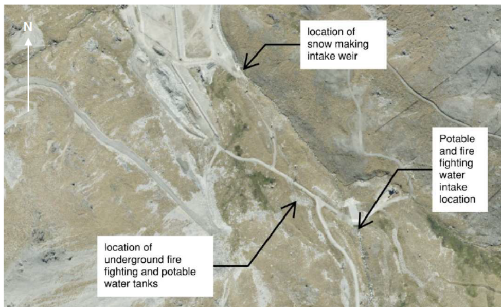
Figure 3: Location of existing water intakes in the Rastus Burn Creek
