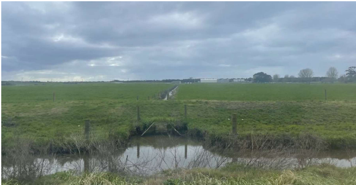
Figure 5: Typical Farm Drain Connecting to Bell Road Drain, with One-Way Valve
