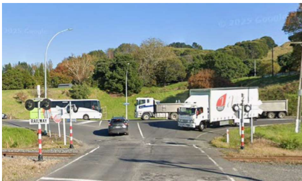
Figure 5-7: Eastern approach FLB (source: Google Maps)
