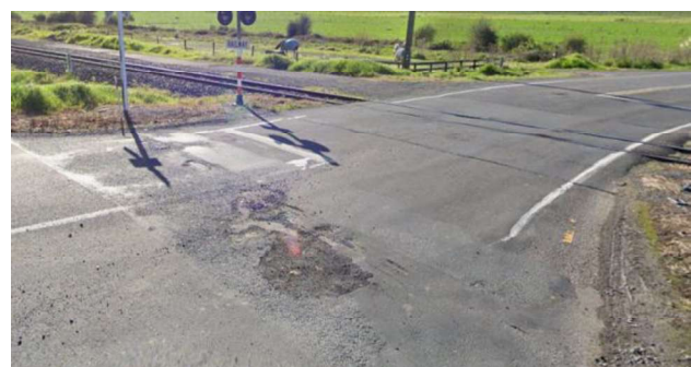
Figure 5-5: Western approach surface rutting (source: Google Maps)
