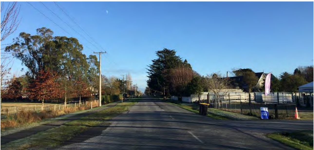
Figure 4: Mill Road Looking West
