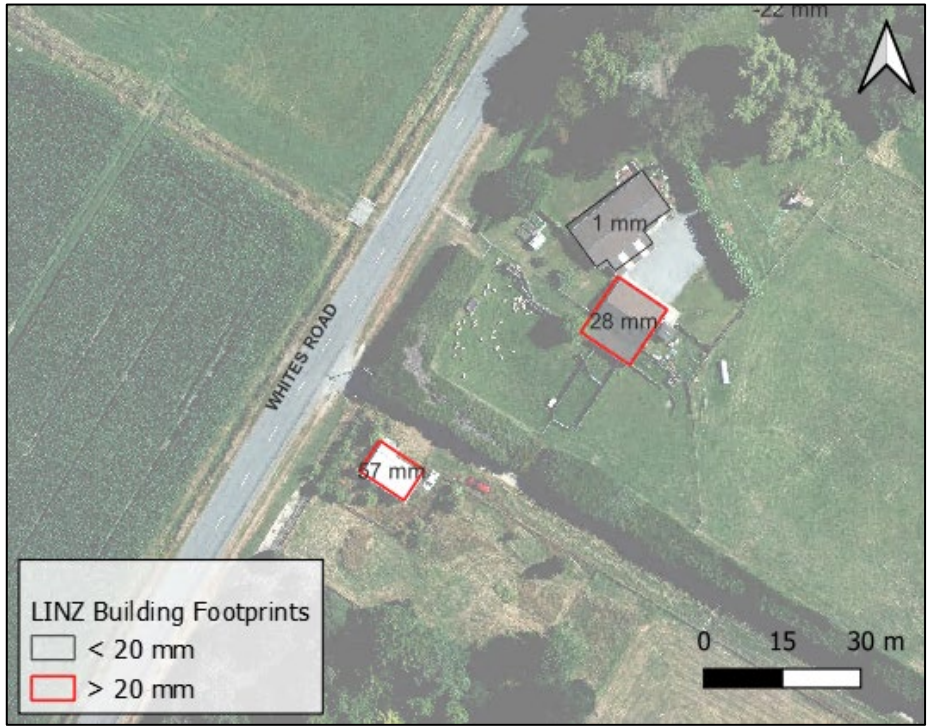
Figure 22: 290 Whites Rd, sheds/garages with flood increase > 20 mm.
