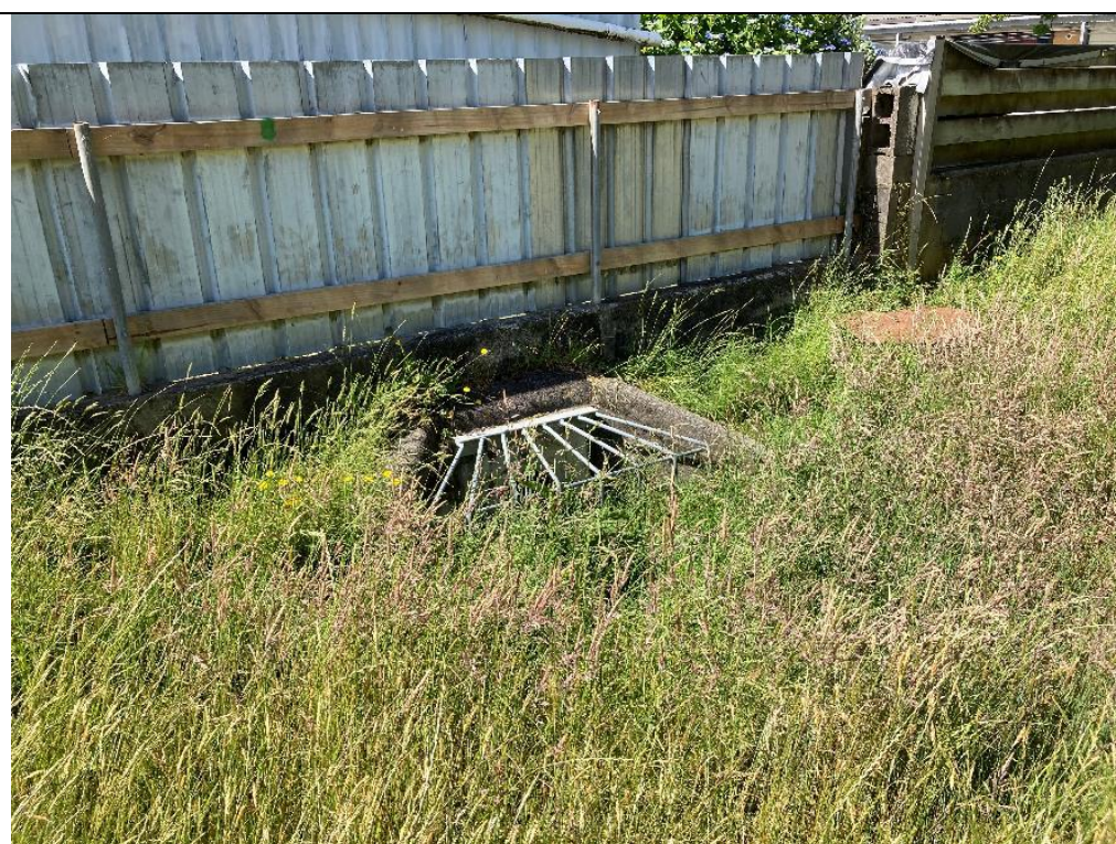
Central southern drain into pipes under residential.
