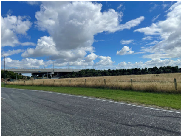
Figure 2: John Paterson Drive looking towards the flyover Springs Road
