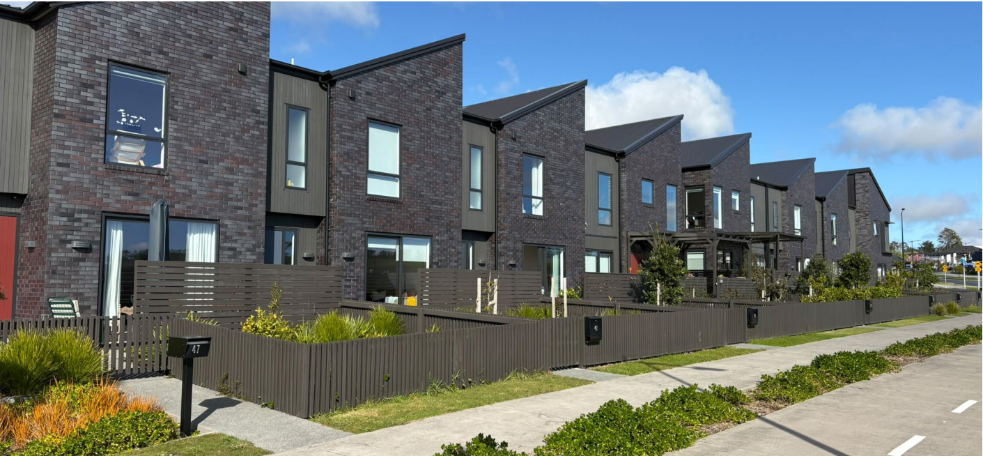
Figure 9 - Low-level landscaping, permeable fencing and screening positioned at the front of a terraced house to deliver on-site amenity and a quality streetscape for terraced housing in Milldale.
