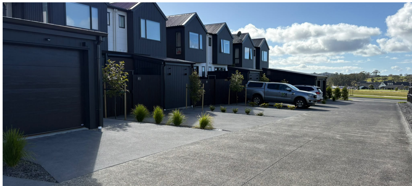
Figure 12 - An existing JOAL in Milldale incorporating material changes and landscaping to delineate parking areas for individual properties.
