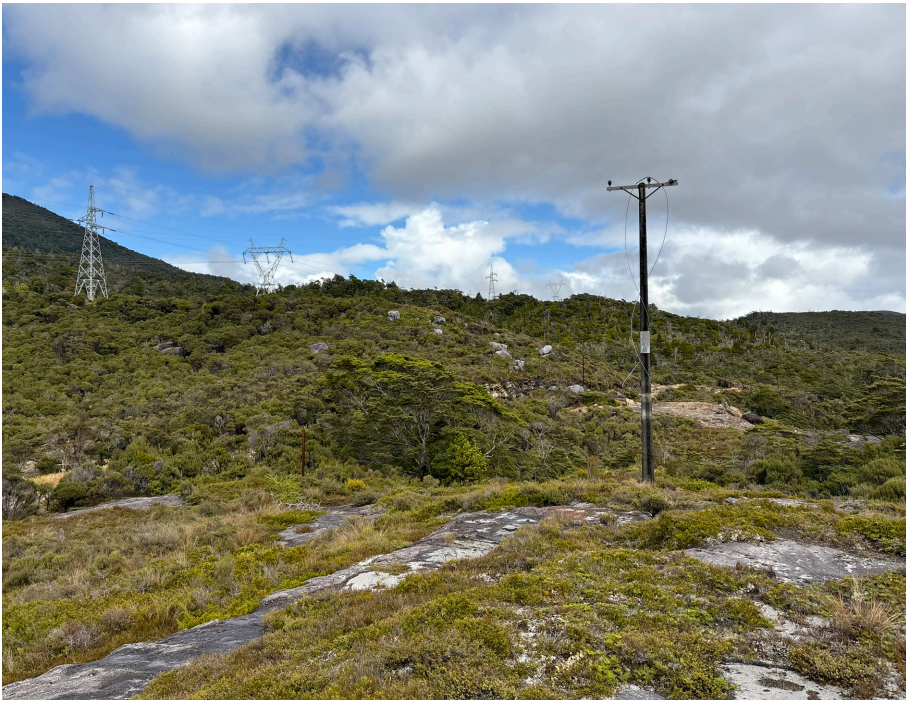
Site Photograph 6: Between the existing Cedar Creek Road and Waimanagaroa River.
