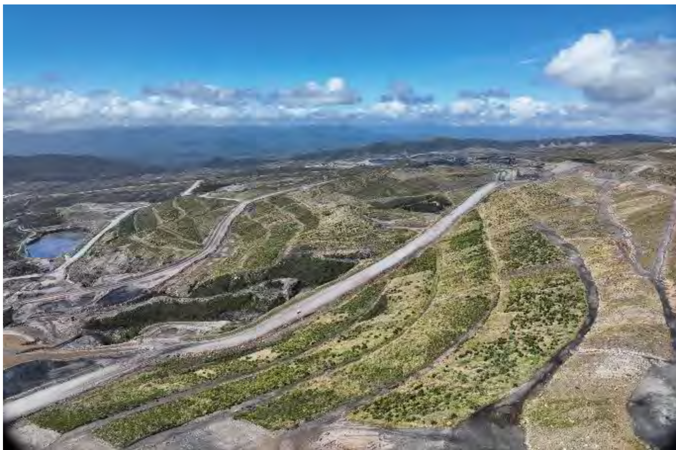
Figure 2-2 Aerial view of Stockton rehabilitation within the Mangatini catchment in February 2026. Mangatini Sump shown to the left of the photo (source: BT Mining)
