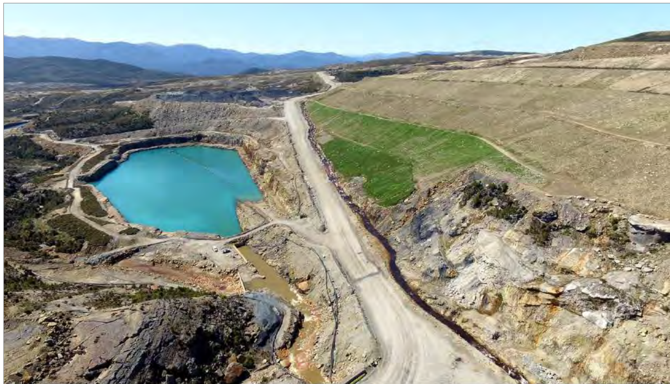
Figure 3-7 Mangatini AMD treatment Sump and rehabilitated landform up-gradient (sources: Solid Energy 2016)
