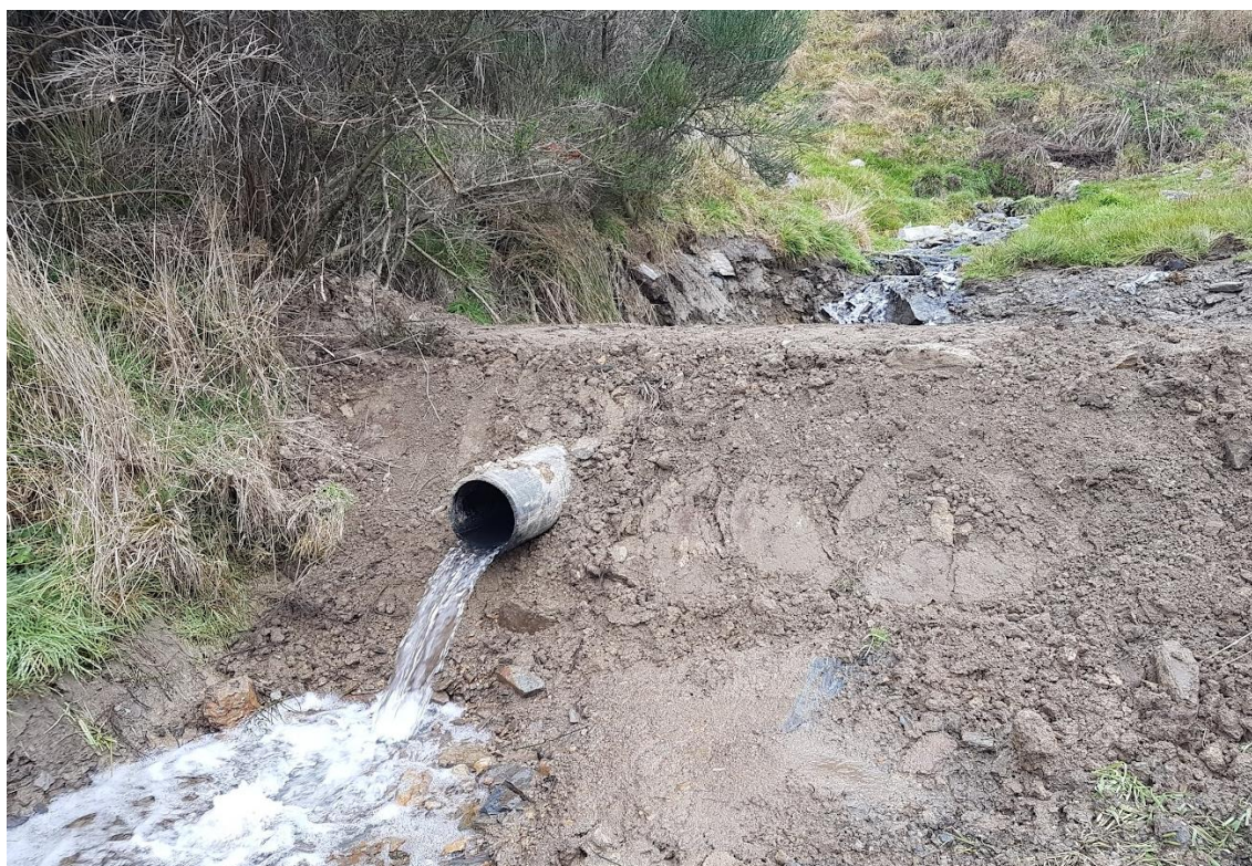
Figure E-2.7 Seepage flow monitoring, Above Murphys Creek silt pond, August 2018.
