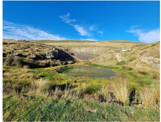
Figure E-2.9 Māori Hen silt pond from embankment (April 2026)
