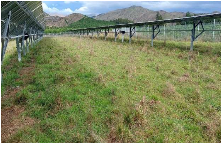
Wairau Valley (Marlborough) field trial solar panel configuration
