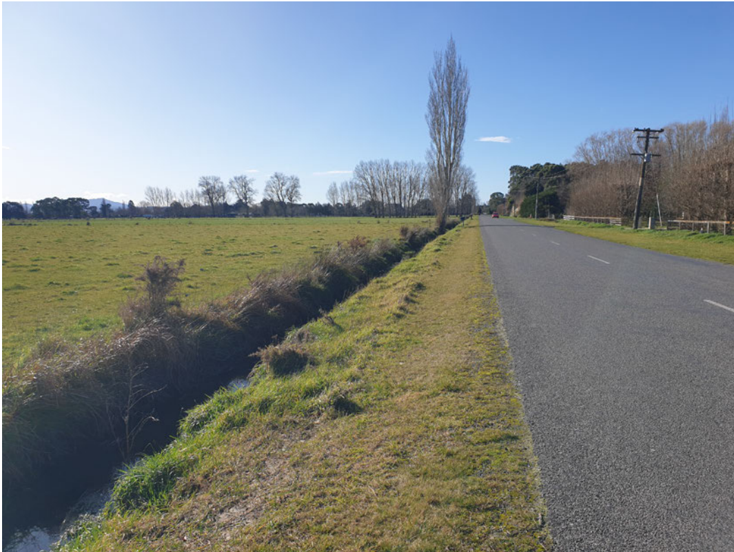
WHITES ROAD - WEST SIDE LOOKING NORTH - NOTE NARROW 'SHOULDER' CLOSE TO DEEP DRAIN
