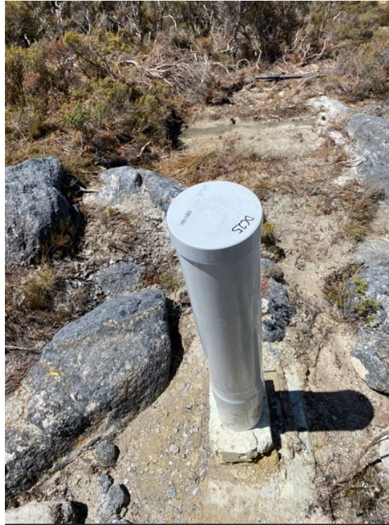
Figure 14: Standpipe installed at Mount Frederick South
