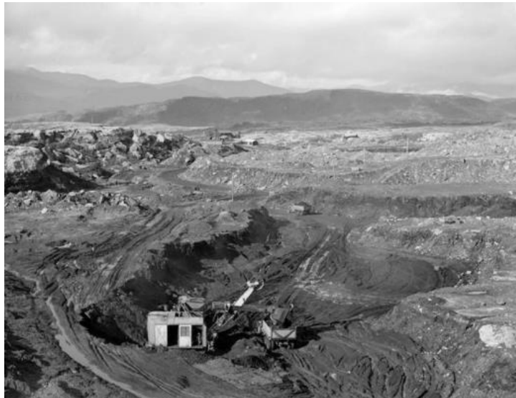
Figure 28: Open cut mining at Stockton, May 1948
