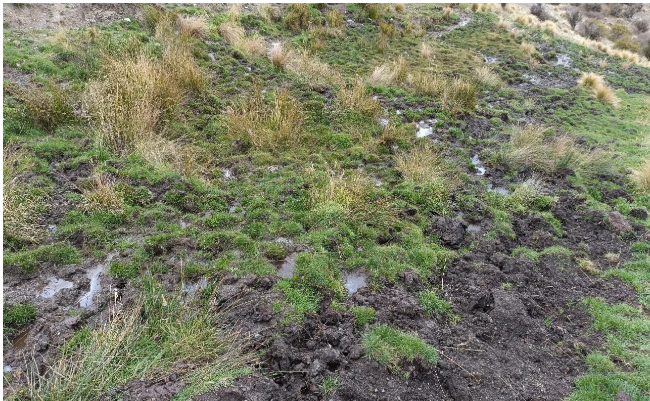
Appendix E3a. A seepage in lower Shepherd's Creek on a hillside.
