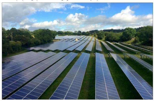
This shows the gaps between photovoltaic arrays allow the water (rainfall) to runoff onto the ground, and that the natural groundcover can remain.
