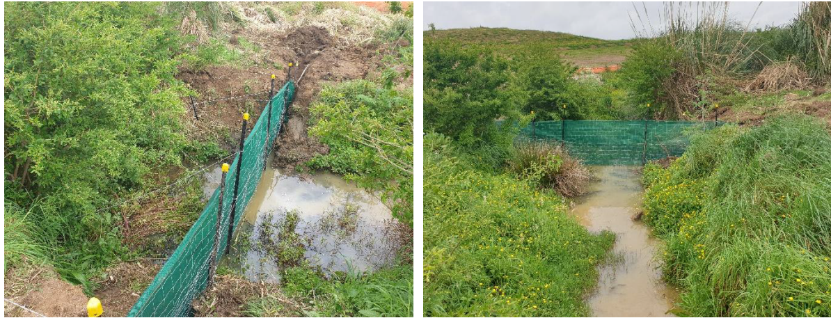
Photo 1 and 2. Photo examples of fish exclusion barriers
