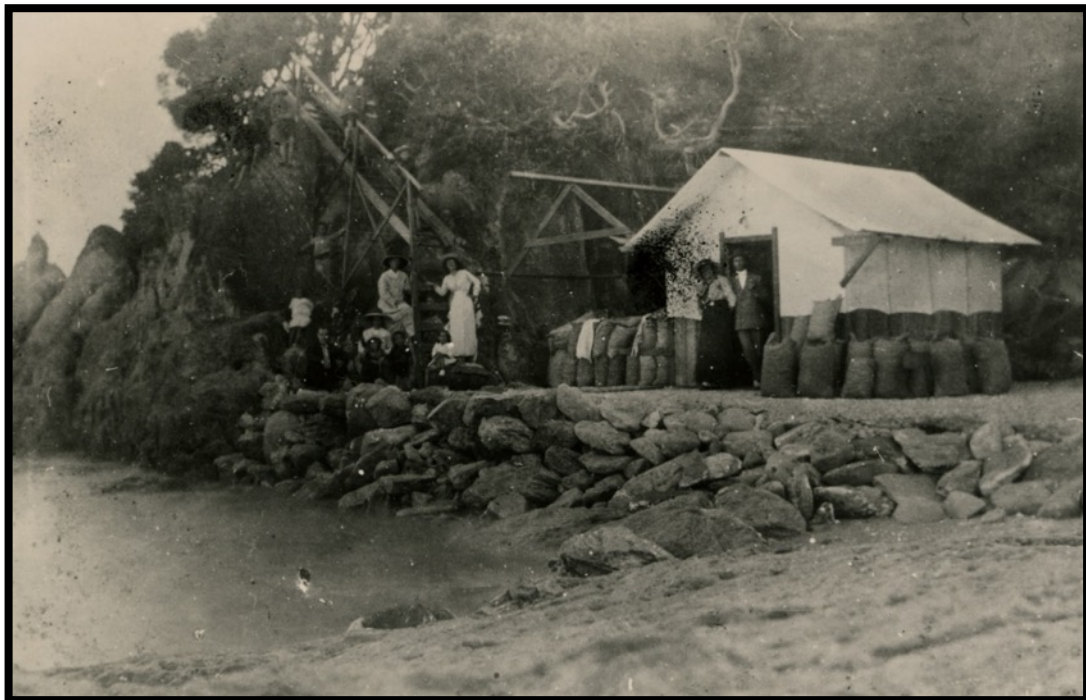
Figure 7: Pilot Bay Stone Jetty, Mount Maunganui, c. 1920s, Tauranga City Libraries, Photo 11-029.
