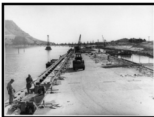
Figure 21: Construction of the first 373 metres of wharf; 1953. From https://www.port-tauranga.co.nz/about-port-of-tauranga/history/
