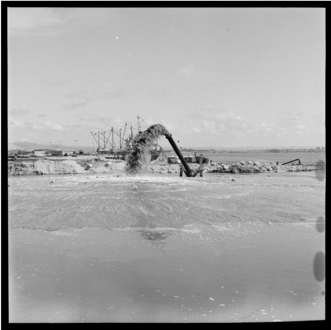
Figure 31: Dredging at Mount Maunganui; 1967. Tauranga City Libraries, photo gca-14825.
