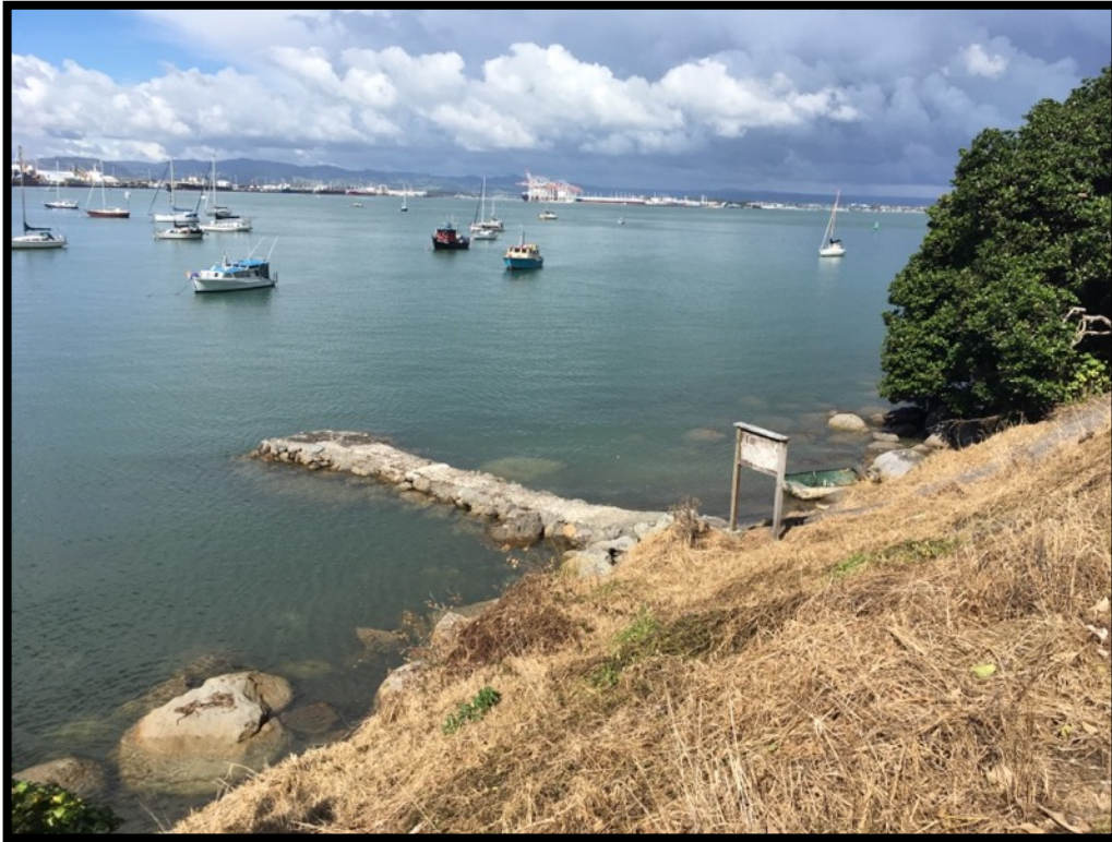
Figure 6: Historic stone jetty, Dr A. McEwan, 17 April 2017.
