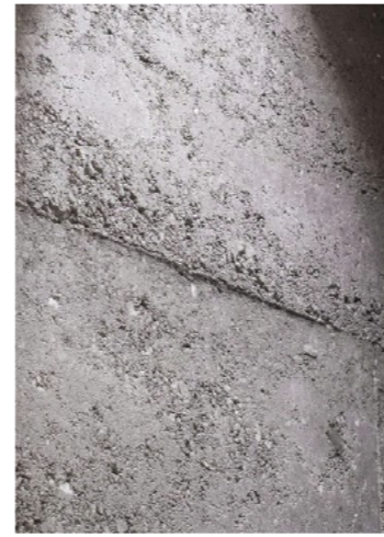
Textured concrete edge walls
