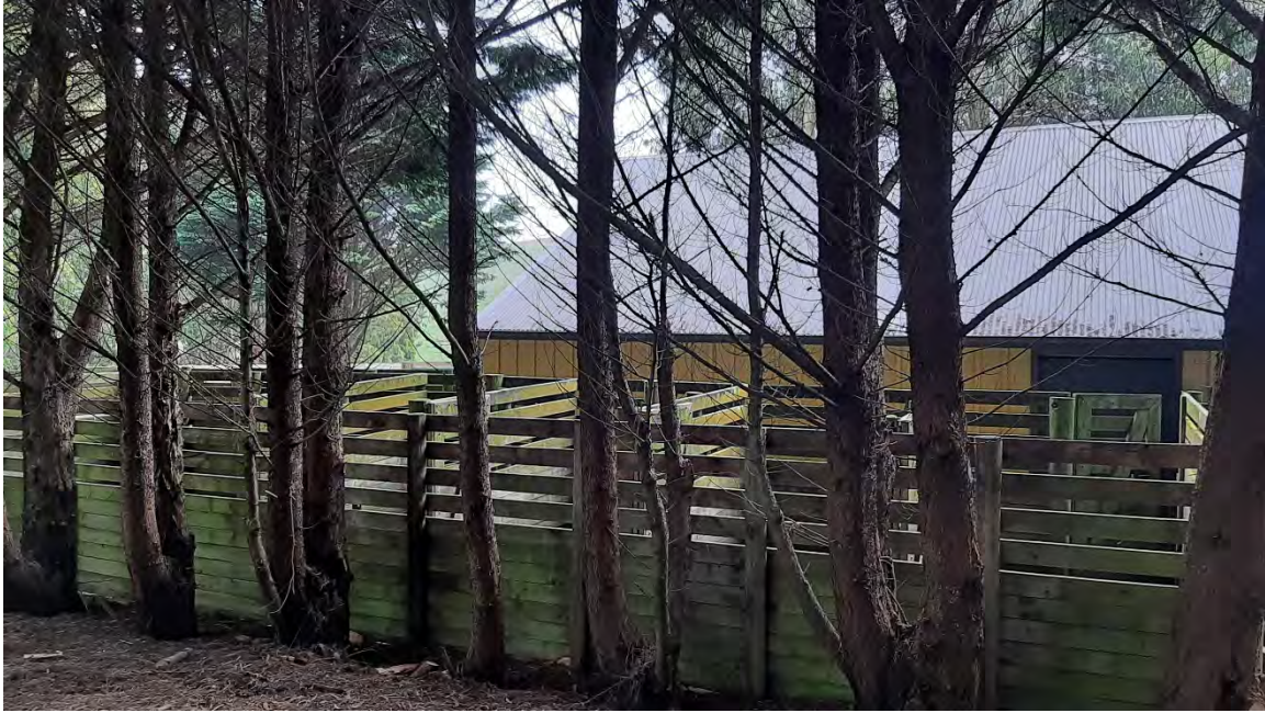
Photograph 3: Rear of this storage shed, showing fenced area where stock are kept.
