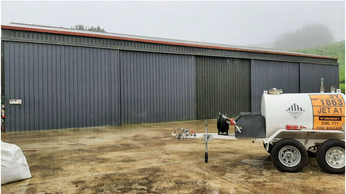
Photograph 11: Storage of Jet A-1 fuel on a mobile trailer visible on the concrete pad of the helicopter hanger. No access was available inside the hanger.
