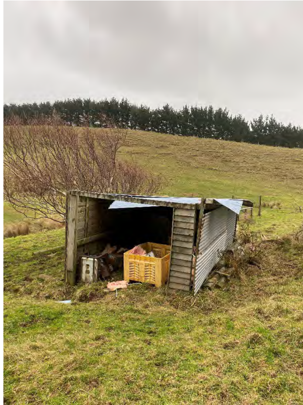
Photograph 3: Storage shed on Part Lot 1 DP 89102 looking northwest.
