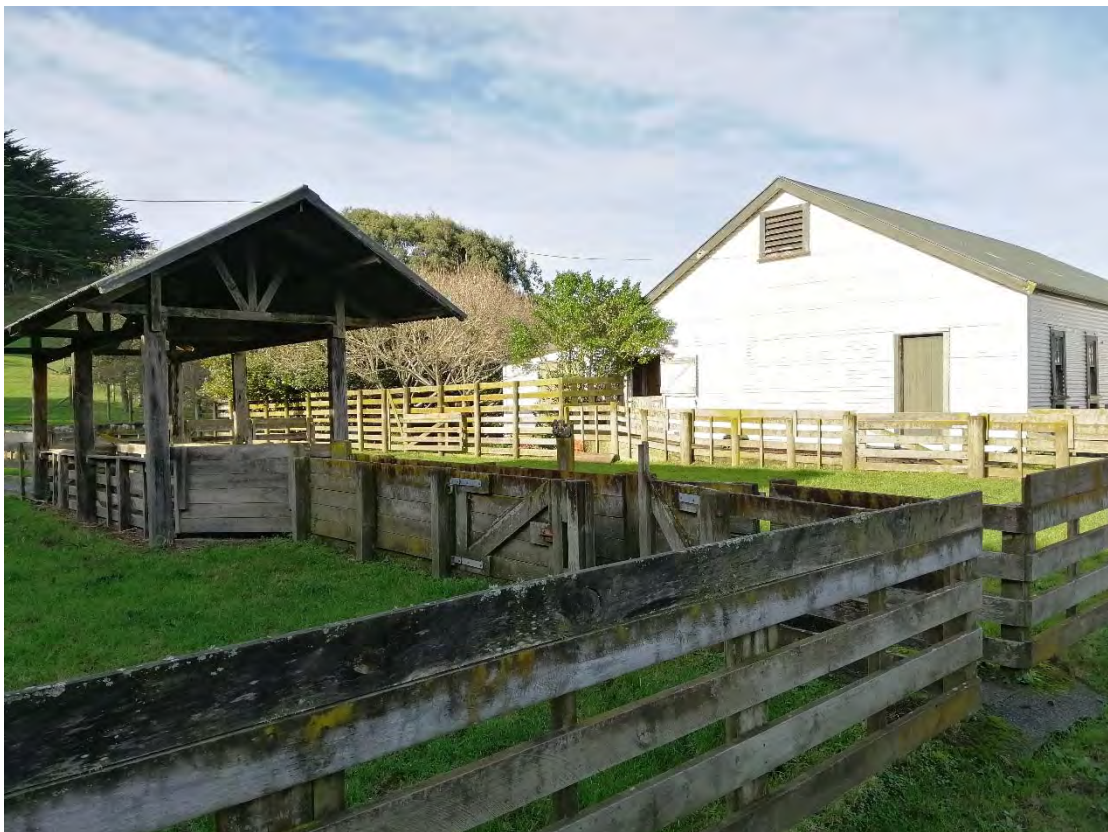
Photograph 2: View looking east of Woolshed and Dock/Race Structure showing sheep yards and concrete pad
