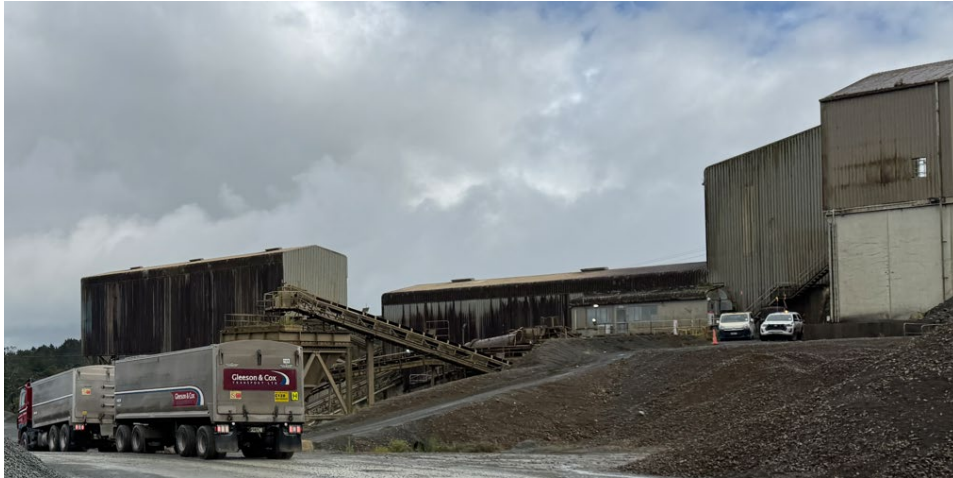
Figure 11: Fixed Processing Plant
