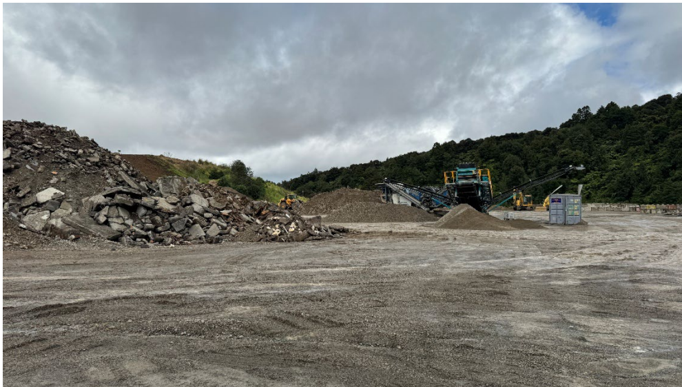
Figure 9: Concrete Recycling Area
