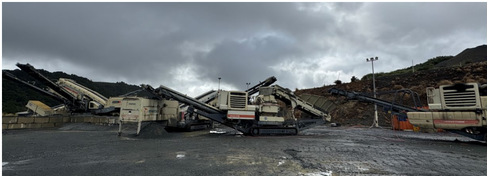
Figure 12: Mobile Processing Plant
