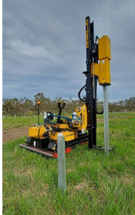
Figure 4.11: Piling machines installing the structures (source: Nova, 2024)
