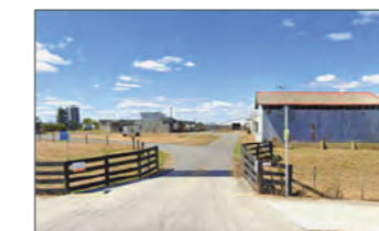
View 'c' Existing entrance to 636 Pencarrow Rd / Te Awa River Ride (West)
