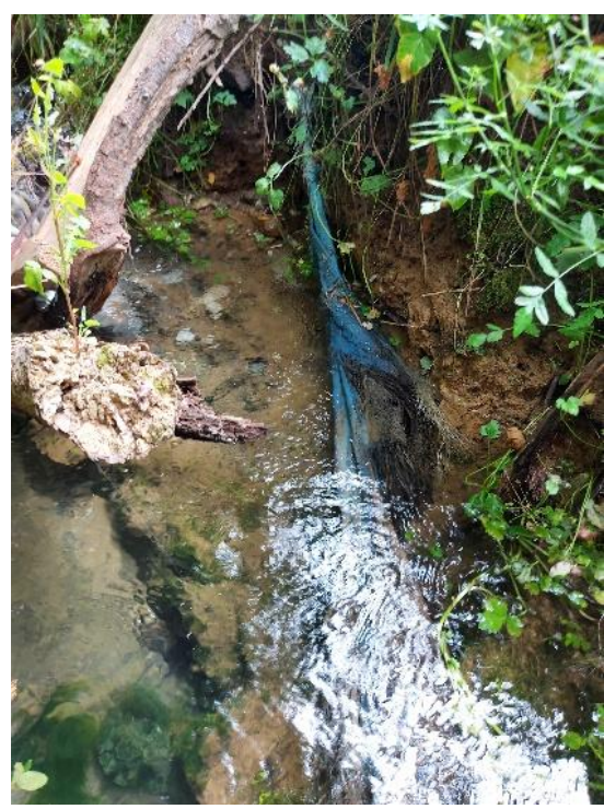
Photo 8: Rubbish debris within channel banks and bed downstream of Pōtea Spring
