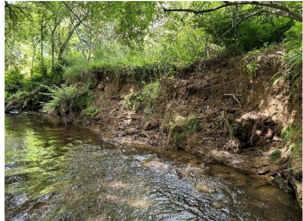
Photo 19: Erosion of Mangawhitikau Stream bank, approximately 20 m upstream of Pōtea Spring. Photograph facing upstream.
