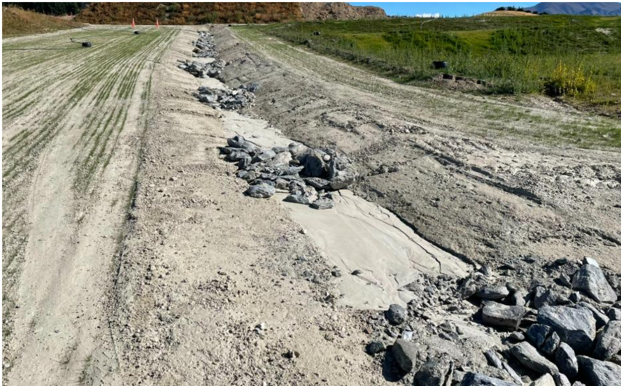
Figure 29: DWDC with rock check dams
