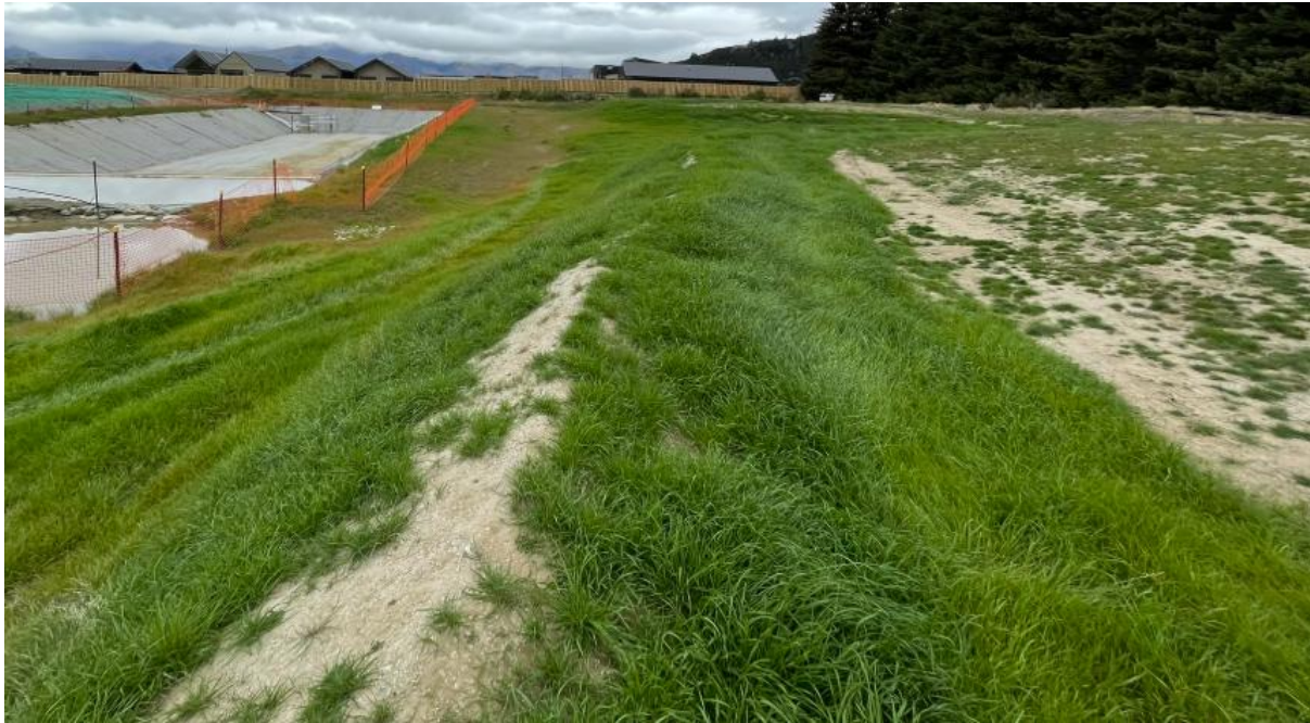
Figure 26: Clean water bund with established grass stabilisation
