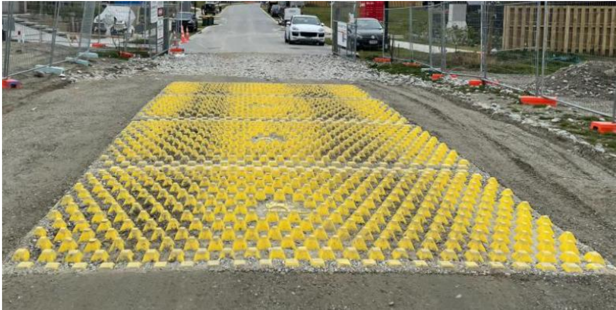
Figure 32: Combination of trackout mats and SCE at site entrance
