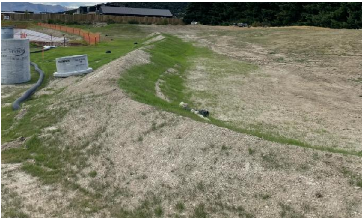
Figure 25: Clean water bund with grass establishing
