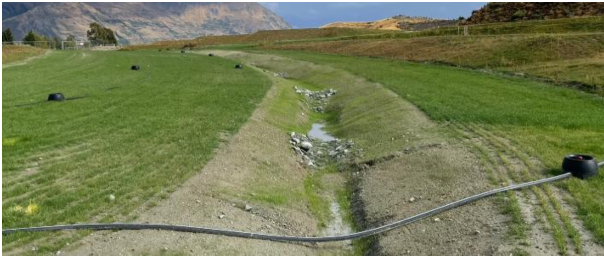
Figure 28: DWDC with establishing direct-drilled grass. When all of the catchment and the channel itself is fully stabilised, it will become a clean water diversion
