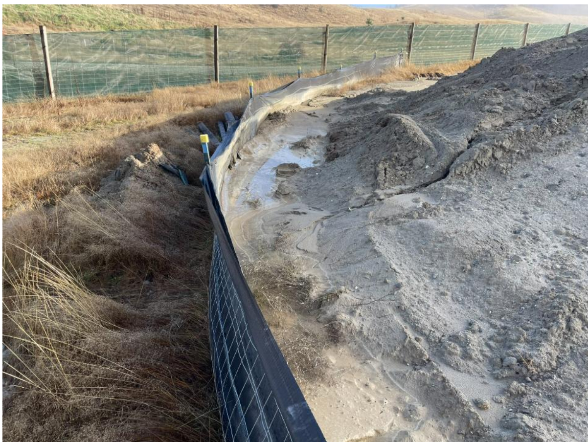
Figure 30: Super silt fence treating dirty upslope water
