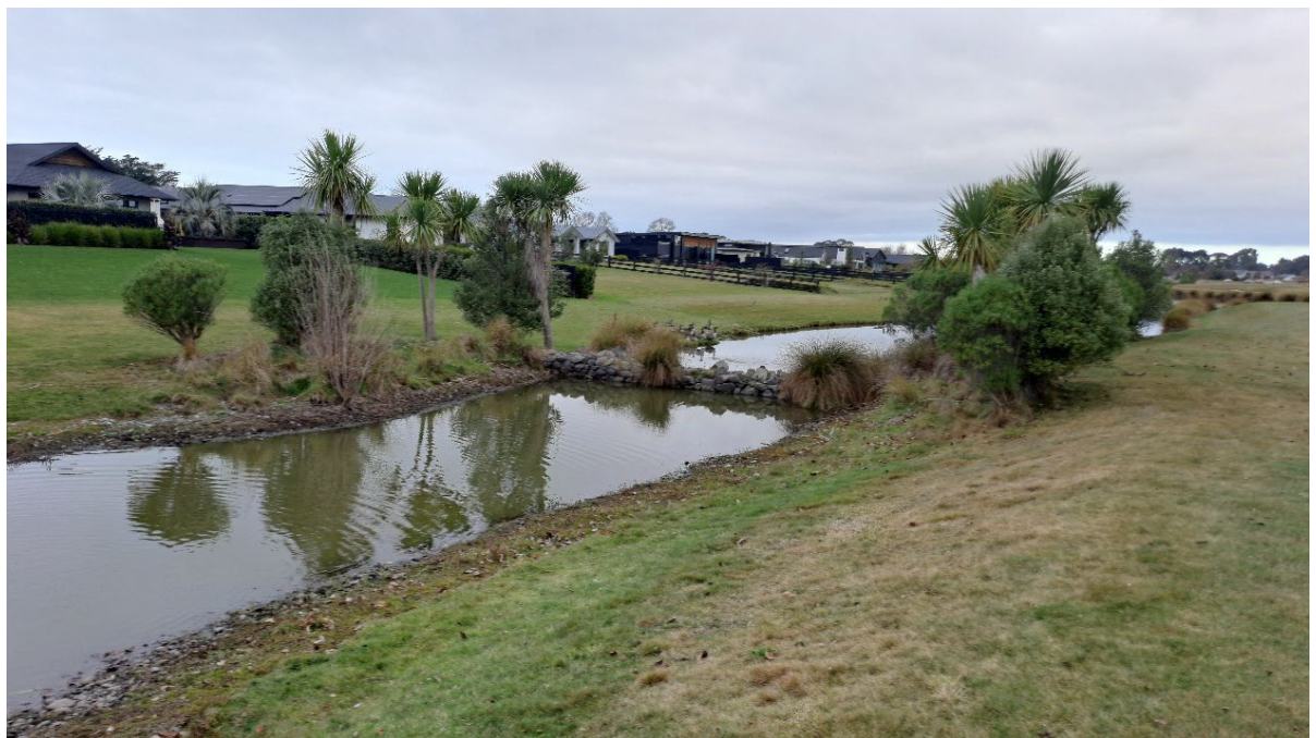
Photograph 22: Channel and rock wall between Pond 5 and Pond 6 (facing north)
