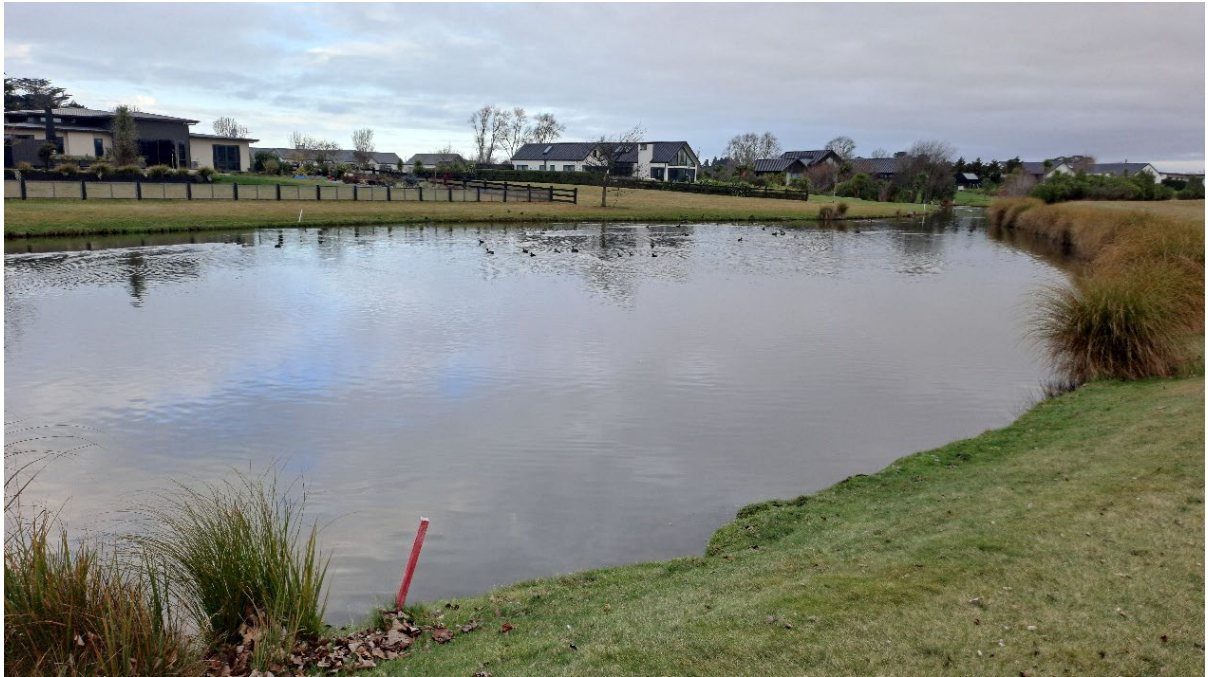
Photograph 21: Pond 5 (facing south)
