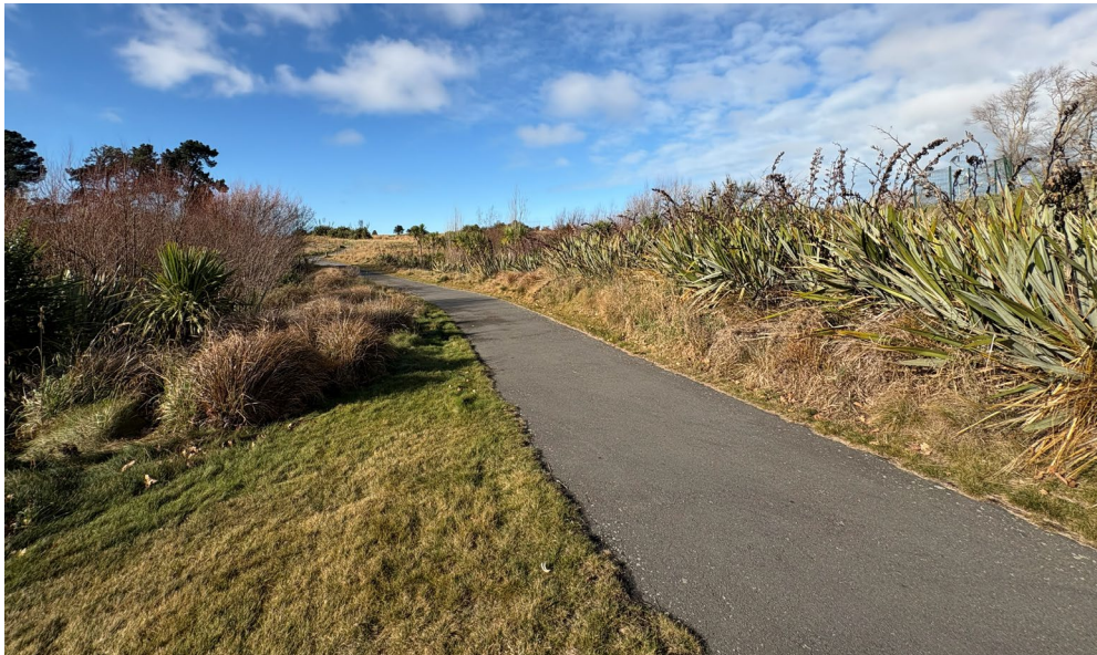
Figure 10: Taerutu Stream is culverted between Wetlands W2 and W3 between Development Areas E and F.
