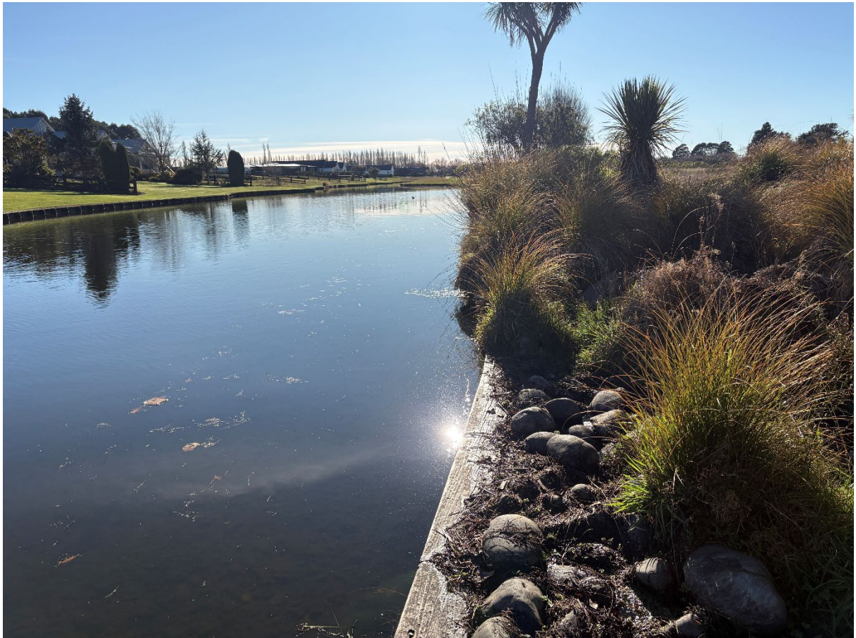
Photograph 25: Pond 17 showing wooden siding around entire perimeter (facing north)
