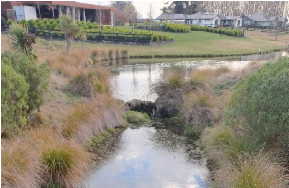
Figure 11: Rock weir between constructed ponds CP1 and CP2
