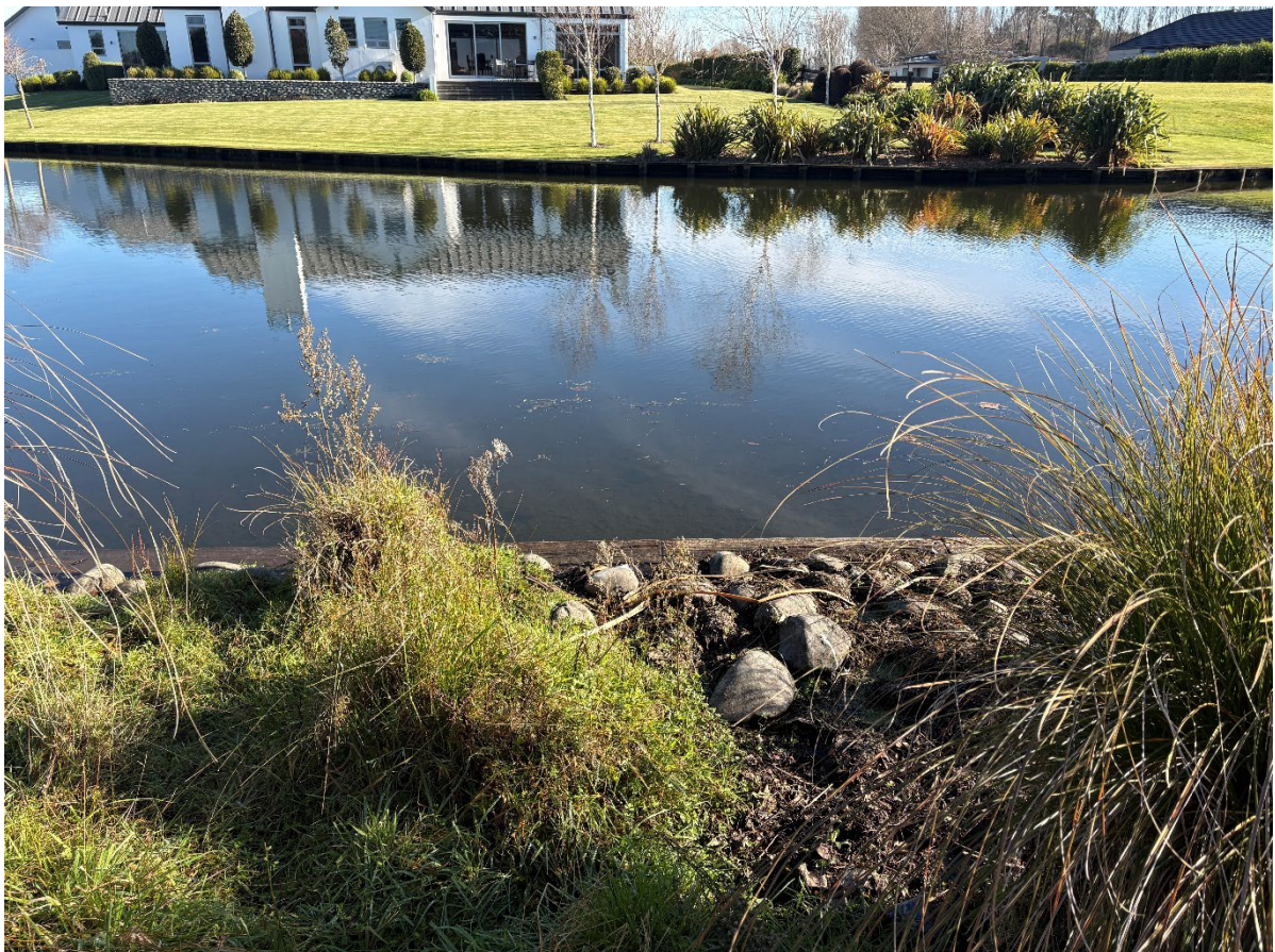
Photograph 26: Spillway between Pond 7 and Wetland 2 (facing west)
