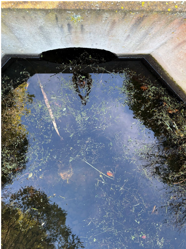
Figure 16: Small diameter culvert under a residential road between Development Areas D and E, connecting constructed ponds CP4 and CP7
