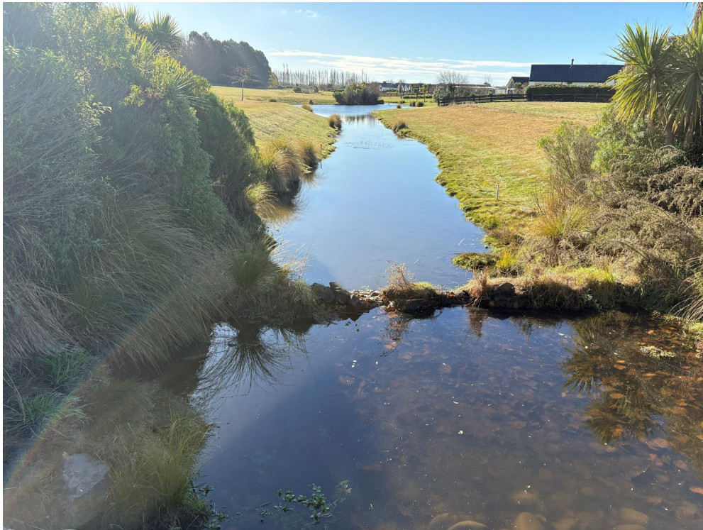
Figure 13: Rock weir between constructed ponds CP3 and CP4
