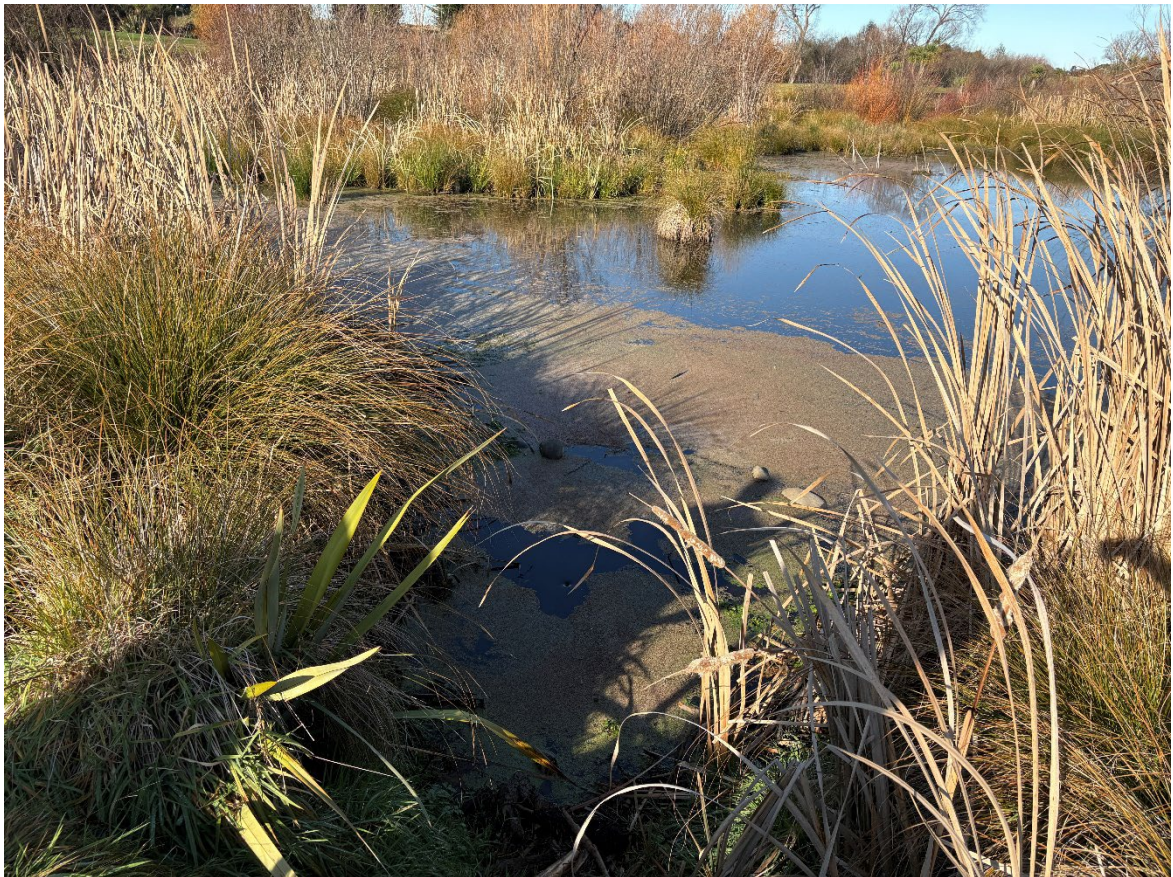
Photograph 42: Wetland 1 (north end) showing orifice weir that connects to Taranaki Stream (facing northwest)
