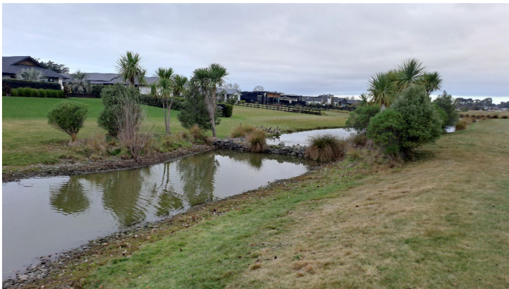
Figure 14: Rock weir between constructed ponds CP4 and CP5
