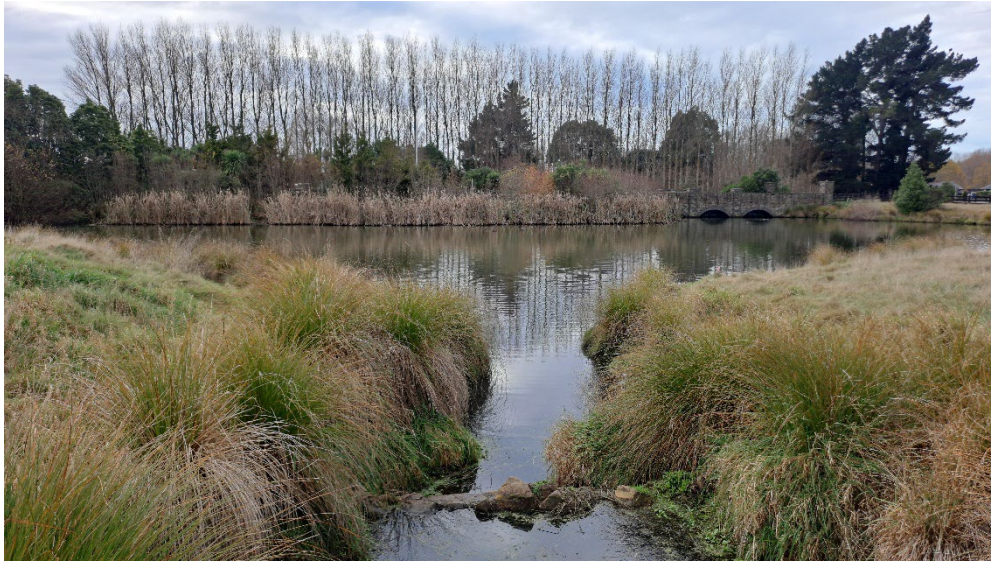
Figure 15: Stepped rock weir system between constructed ponds CP9 and CP10 in Development Area A.
