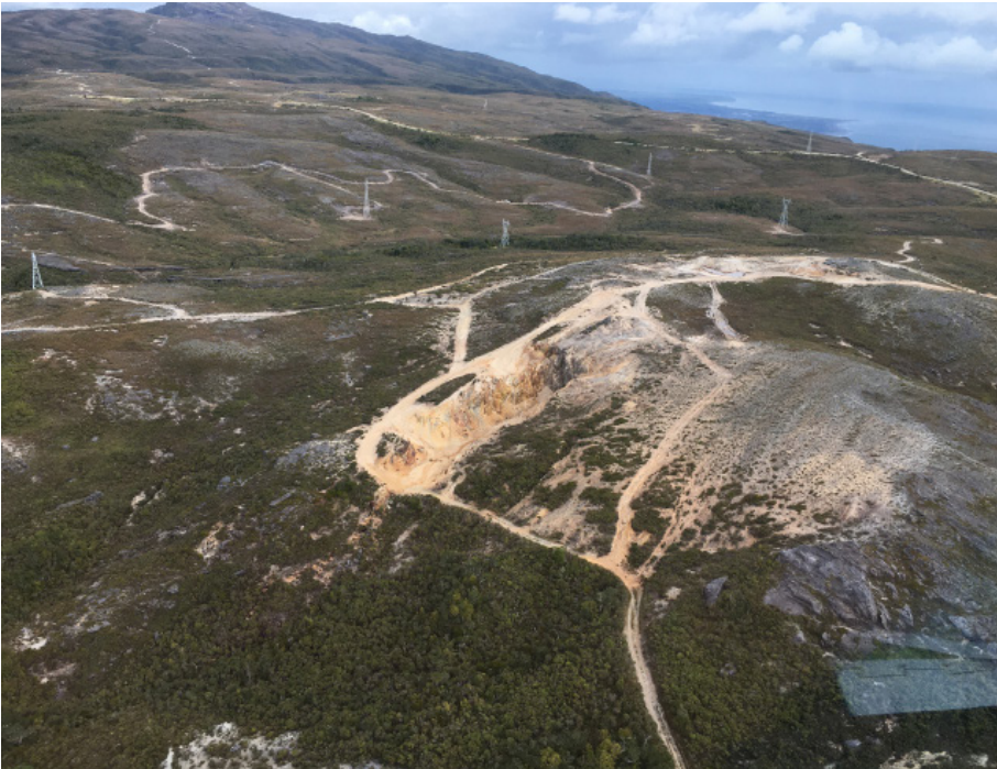
Site Photograph 13: Looking south west.
