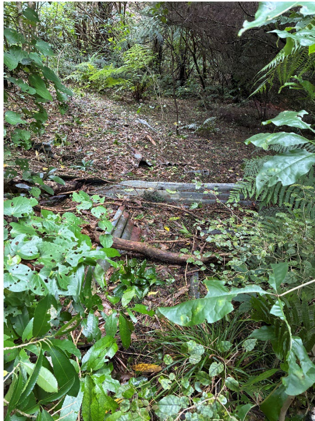
Photograph 8: Example of metal sheeting at SS03 and SS04.
