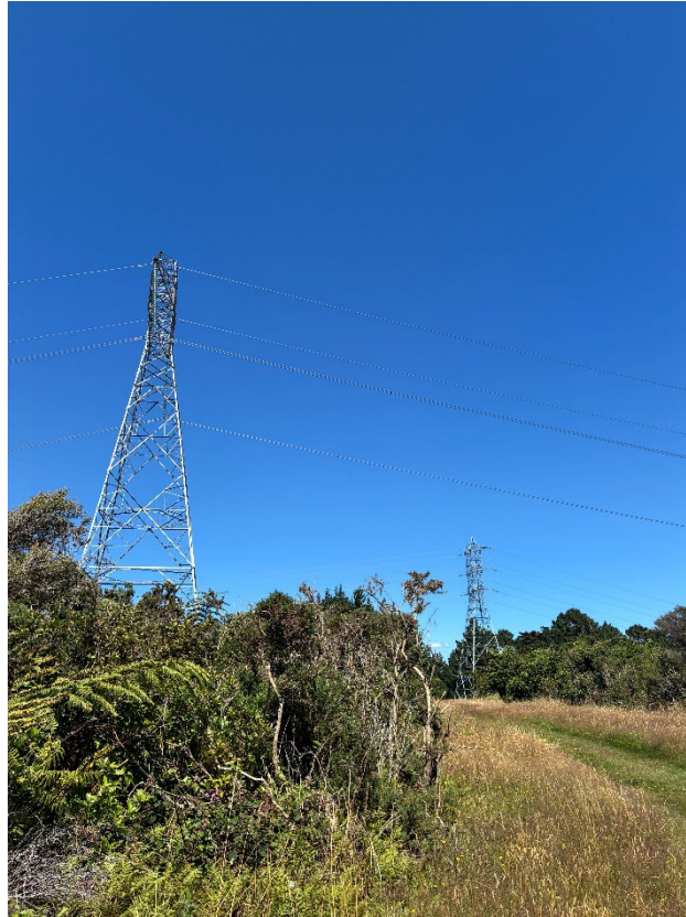
Photograph 1: View of onsite pylons, looking north.
