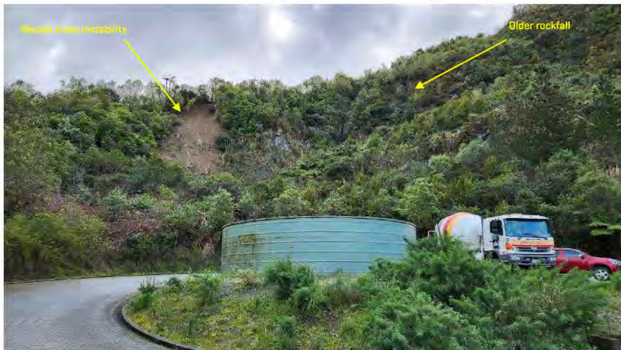
Figure 5-2: Remnant quarry batters Firth Block
