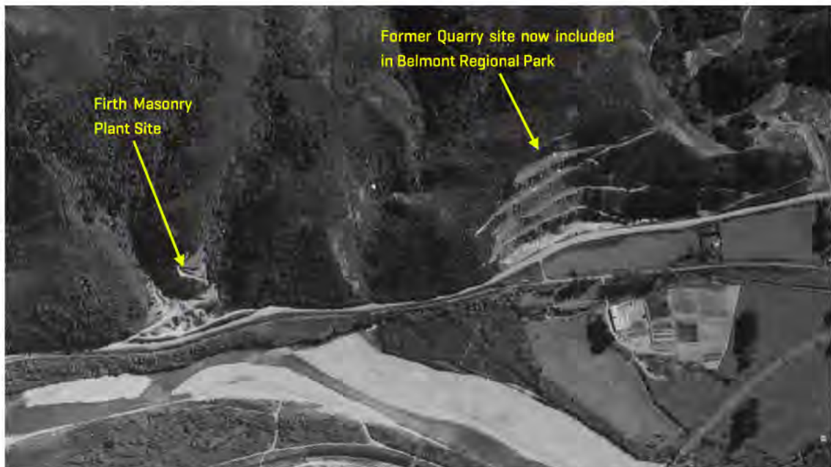
Figure 5-6: 1957 aerial photograph illustrating historic quarry faces incorporated in Belmont Regional Park.
