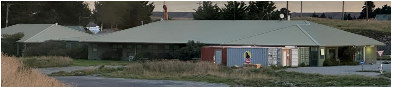
B2.2: Main Office (Building mounted security lights)
