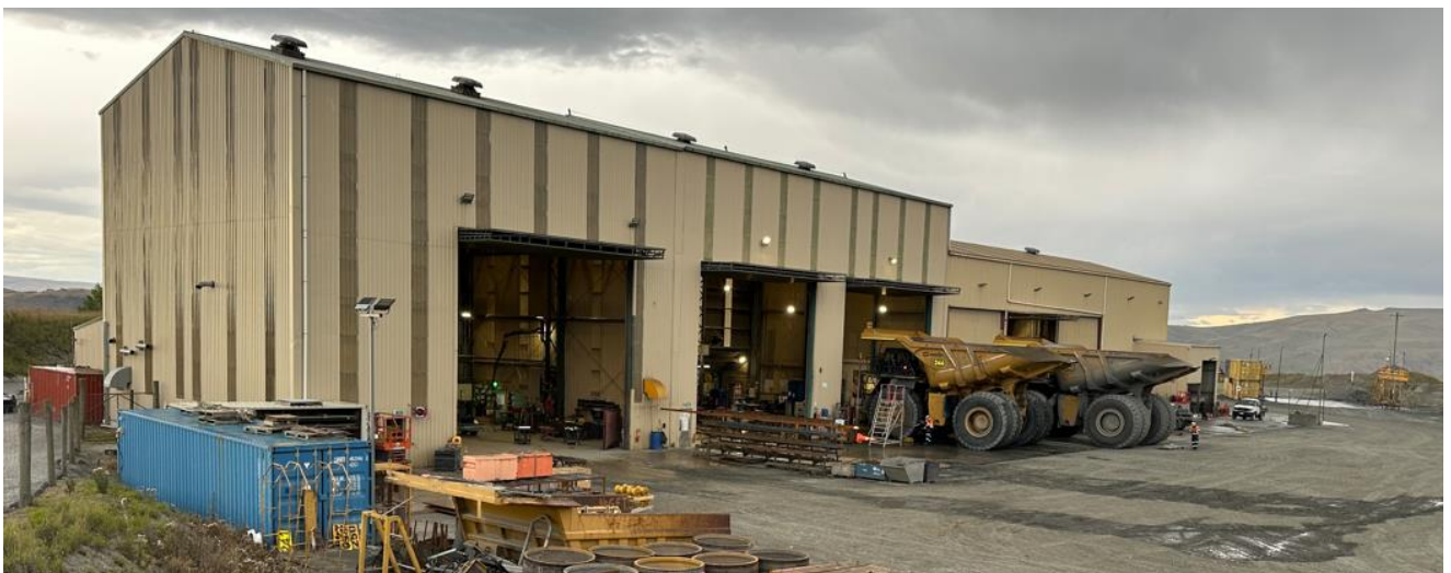
B2.6: Existing Open Pit Maintenance Workshop (Mainly building mounted lights)
