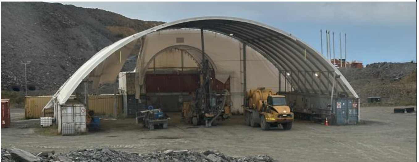
B2.8: Coronation Maintenance Igloo Workshop (Mainly building mounted lights)
