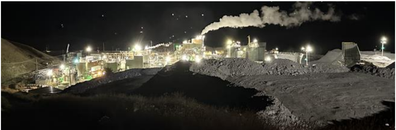
B5.7: Processing Plant
