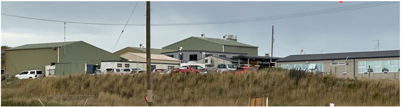
B2.5: Underground Maintenance Workshop (Mainly building mounted lights)
