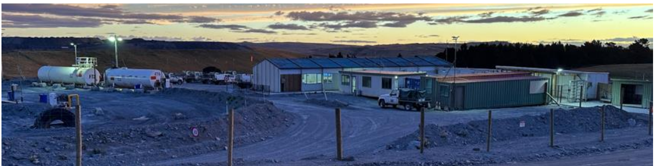
B2.3: Open Pit Office and Parking (Building mounted security lights. Column mounted parking lights)
