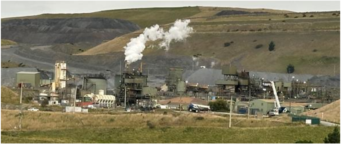
B2.4: Processing Plant (Mainly structure mounted lights)
