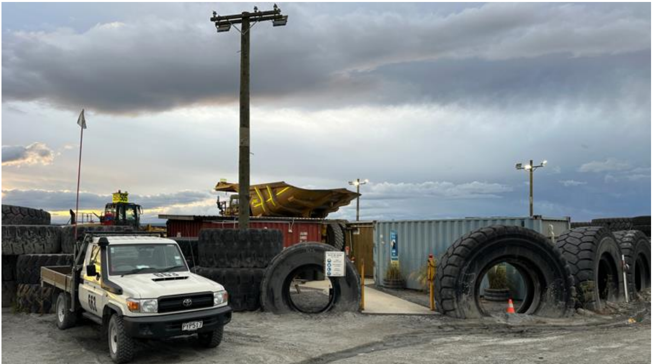
B2.7: Existing Tyre Maintenance Yard (Column mounted lights)
