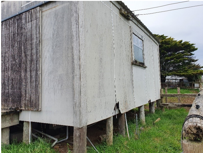
Stables (2) - Minor Damage to PACM Cladding
